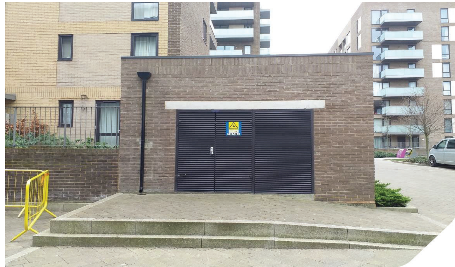
Photo 02: Electricity substation in development next to Braithwaite Park
