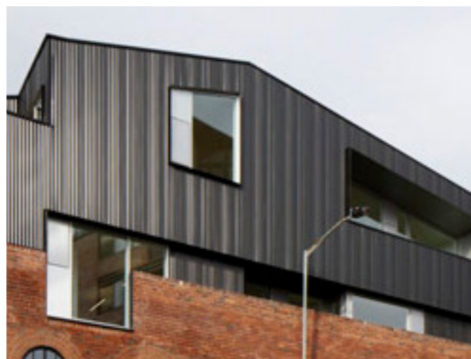
Fig.383 Contrasting building top with playful roof form
