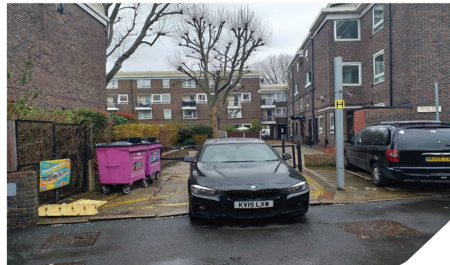
Photo 18: Four storey flats of the development between Abbot Road and Nairn Street
