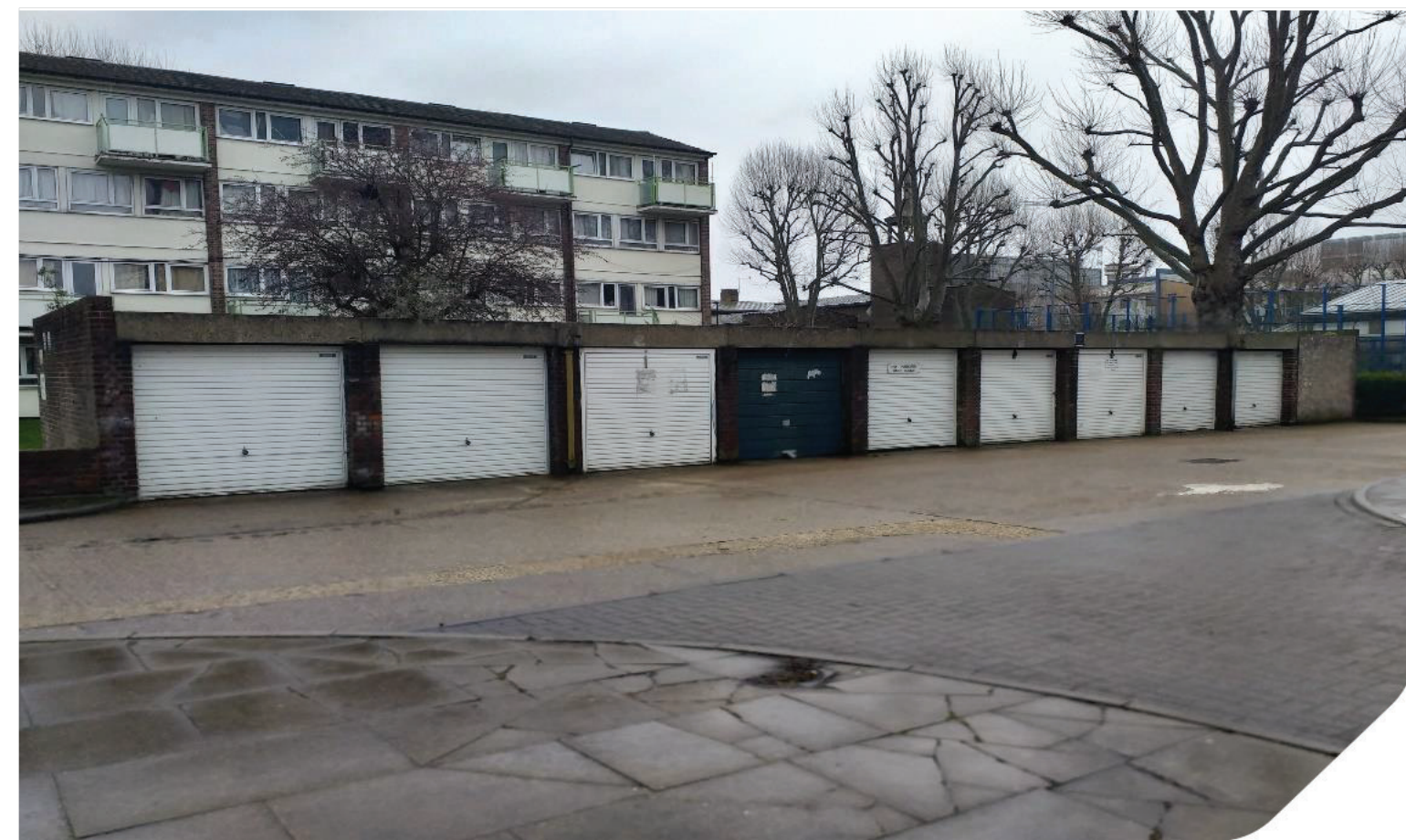
Photo 17: Row of domestic garages off Ettrick Street
