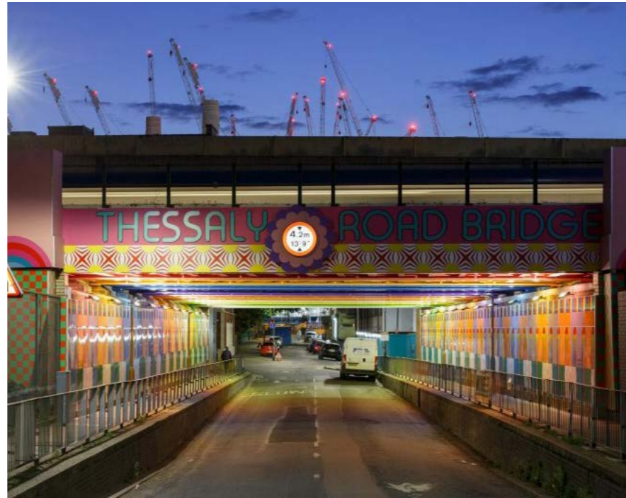
Fig.544 Distinctive character and welcoming fun lighting to Underpass
