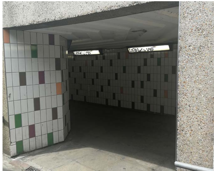
Fig.540 View into the pedestrian underpass
