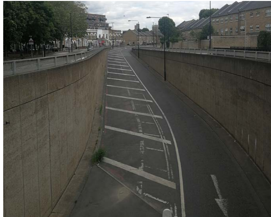
Fig.539 View from the A12 above the vehicular underpass
