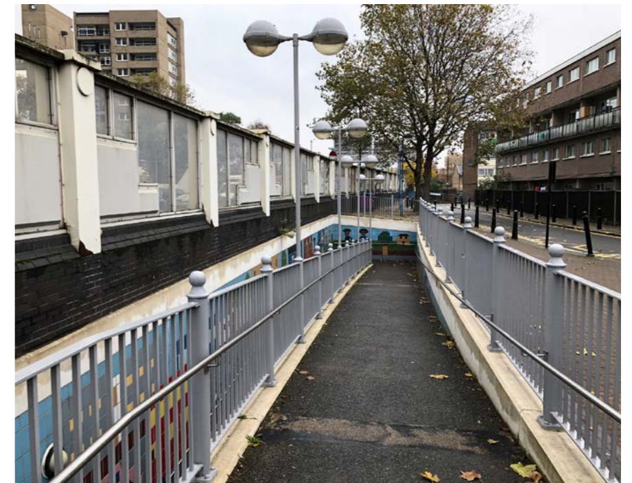
Fig.644 1:10 sloped access to the Pedestrian underpass
