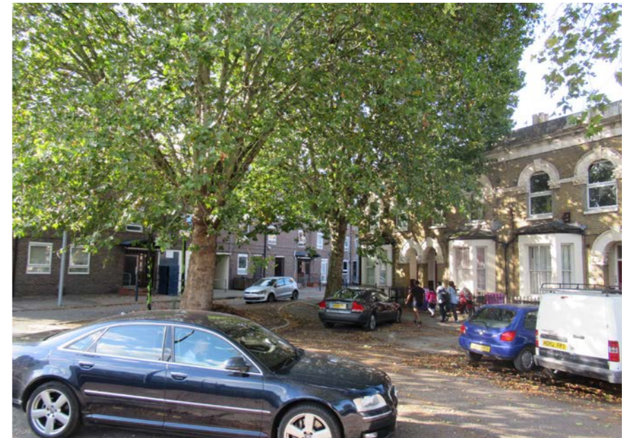
12 Fig.42 Nairn Street estate and terraced houses along Abbott Road
