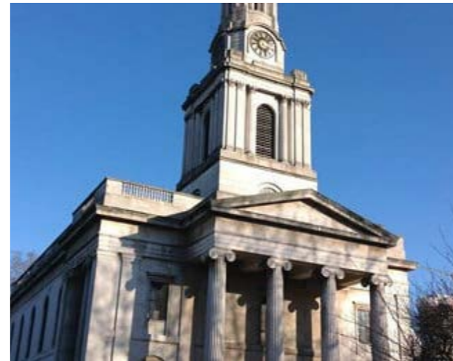
12 Fig.115 All Saints Church with St Frideswide: Grade II listed church built in 1817 and designed by J Hollis
