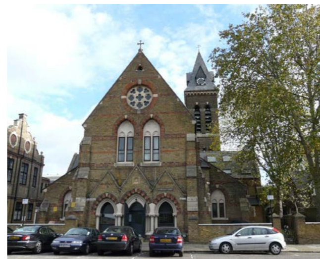
5 Fig.108 Church of Michael and All Angels: A former church which has now been converted into flats, built in 1864 by R.W. Morris
