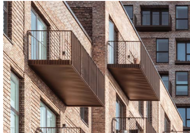
Fig.393 Projecting metal balconies
