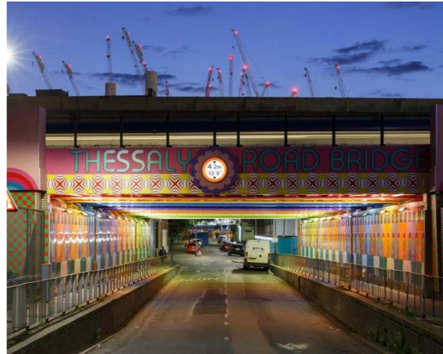
Fig.544 Distinctive character and welcoming fun lighting to Underpass
