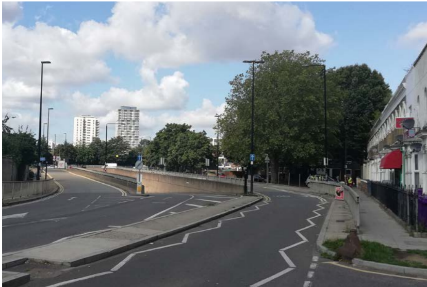
4 Fig.128 Entrance to the vehicular underpass on Abbott Road allowing northbound egress onto the A12. This creates a physical barrier between Aberfeldy Estate to the south and Nairn Street Estate to the north making pedestrian movement extremely difficult.
