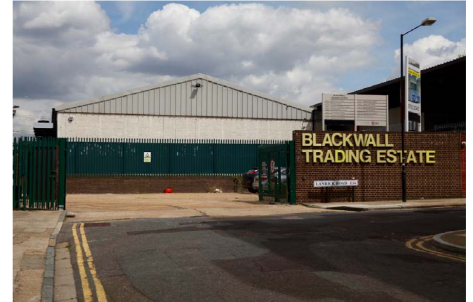
3 Fig.92 Blackwall Trading Estate comprises of single storey industrial units and warehouses with first floor ancillary offices and open yard space
