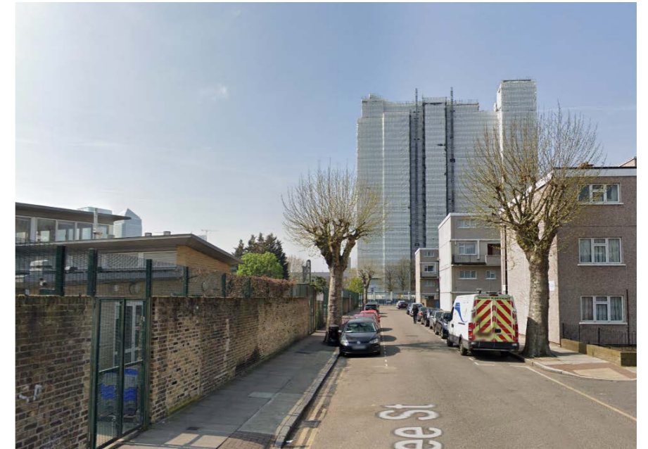
3 Fig.33 View along Dee Street to Balfour Tower
