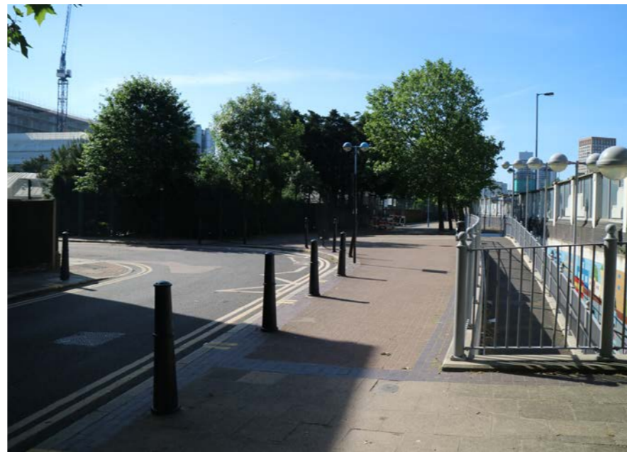
5 Fig.35 Dee Street pedestrian underpass
