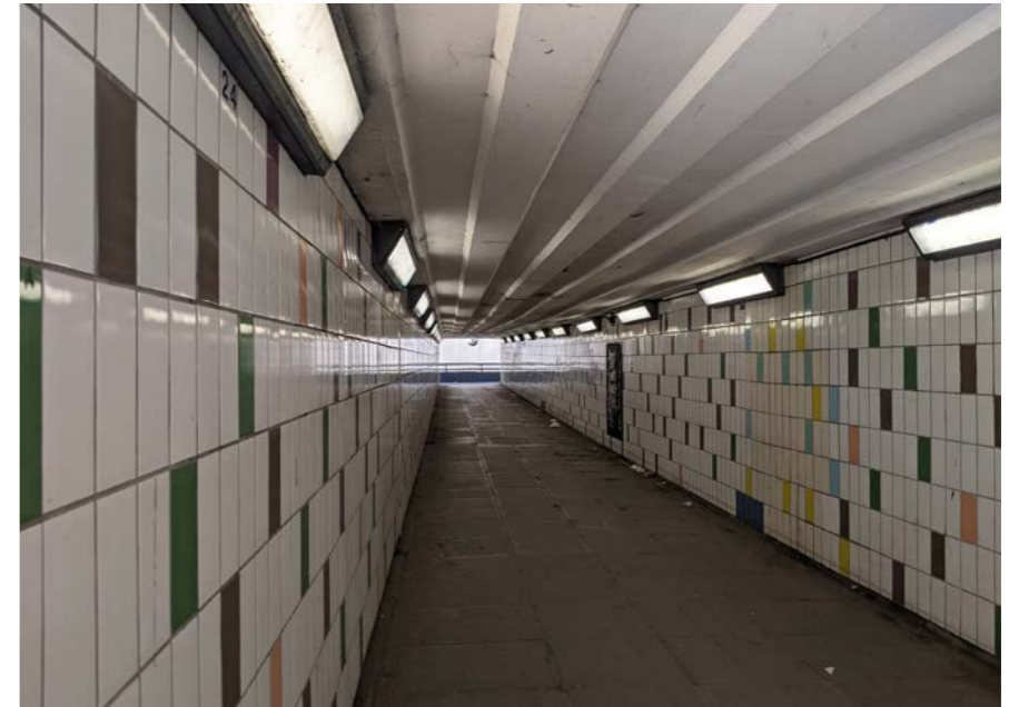
9 Fig.39 Pedestrian underpass under the A12
