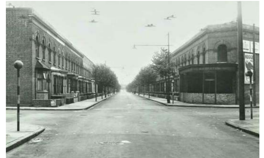
Fig.15 View along Abbott Road showing traditional terraced housing, some of which remains today
