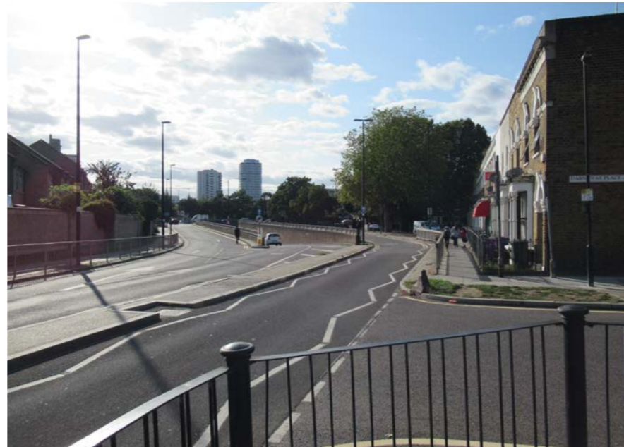
11 Fig.41 Looking west along Abbott Road and the ramp to the vehicle underpass
