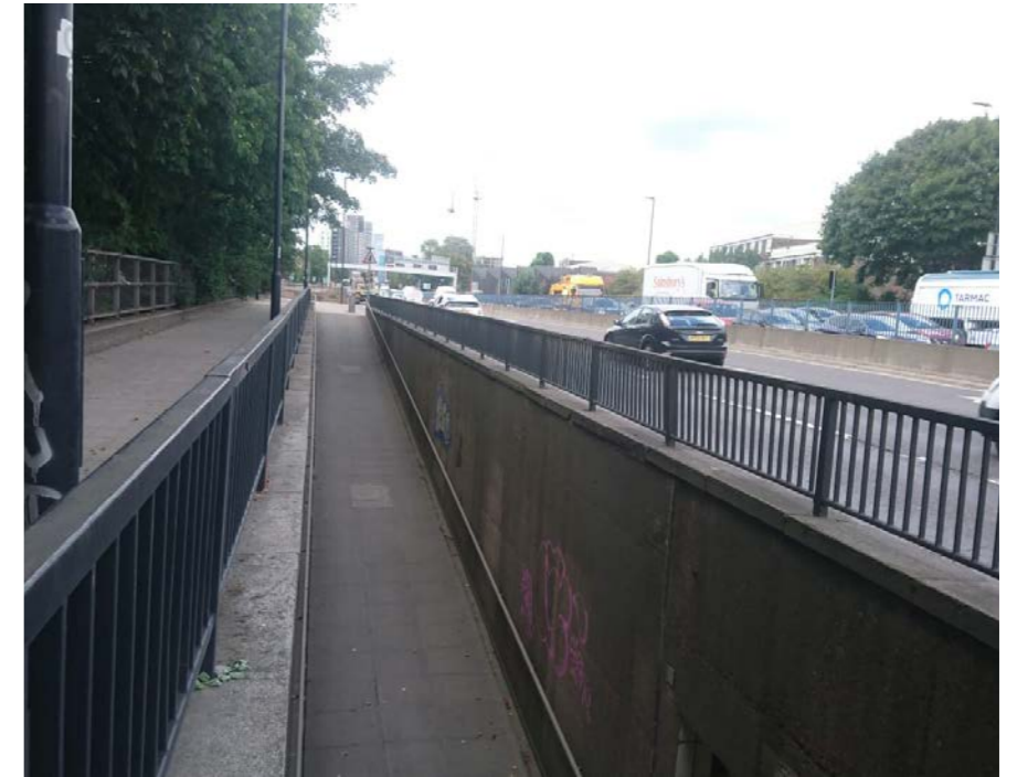
Fig.541 Exit from the pedestrian underpass to Jolly's Green
