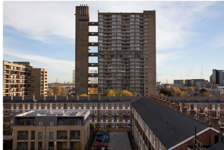
1 Fig.84 Balforn Tower: 27 storeys / up to 84.7m AOD
