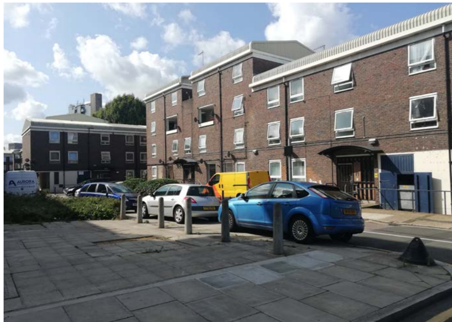
16 Fig.46 Looking south along Nairn Street
