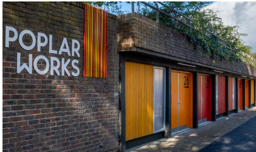
Fig.56 Existing garages converted into small studios
