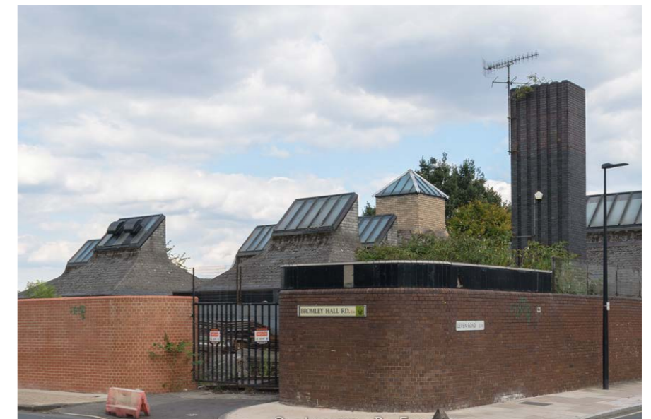
6 Fig.95 Vacant Bromley Hall School, which has the potential to be refurbished and reused
