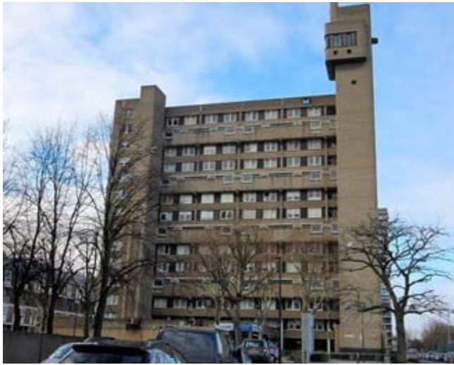
7 Fig.110 Glenkerry House: Grade II listed residential building which forms part of the Brownfield Estate, built in 1977 and designed by Erno Goldfinger
