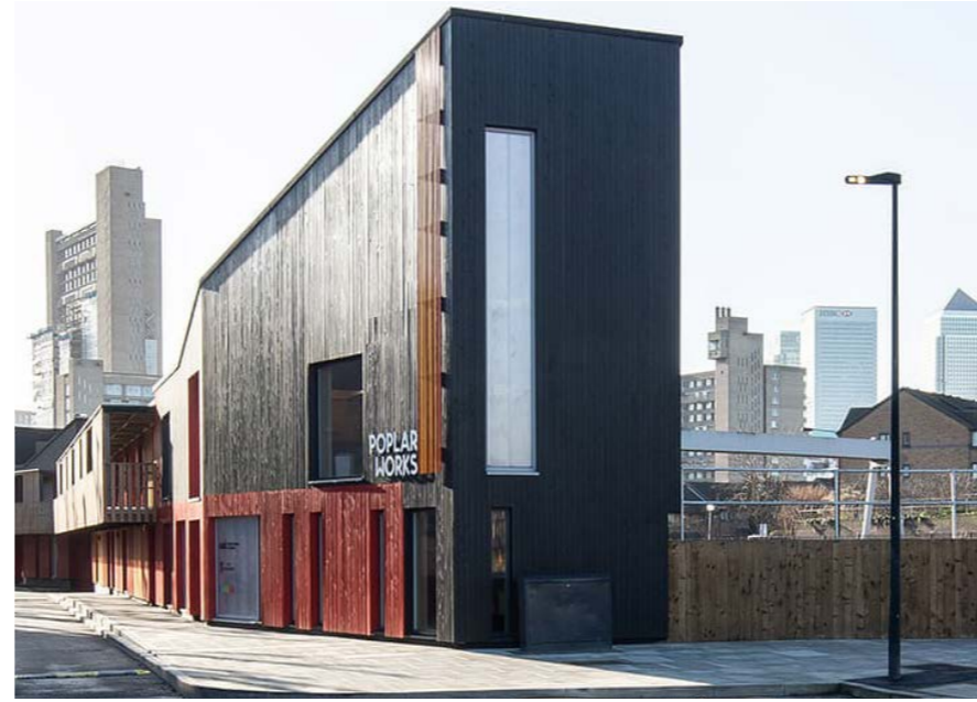
14 Fig.44 Poplar Works development along Nairn Street
