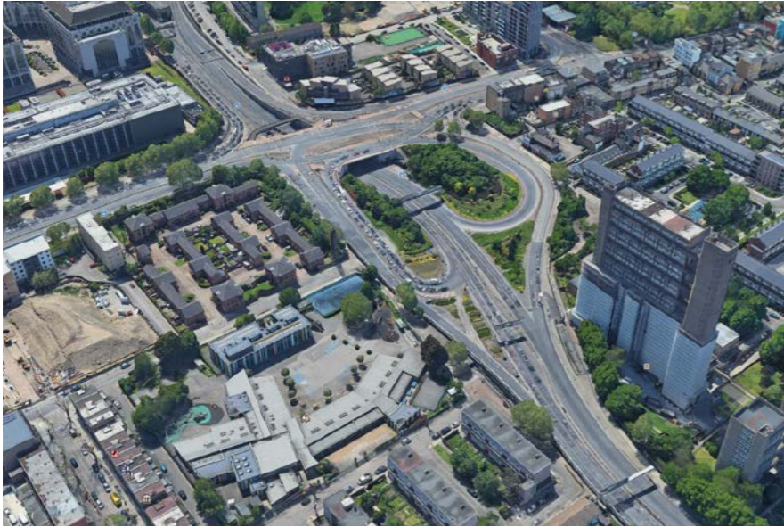
1 Fig.125 Aerial view of the large junction between A12 and A13 towards the Blackwall Tunnel
