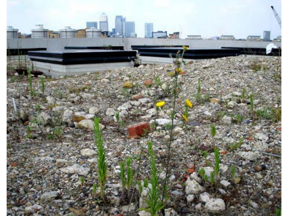
Fig.696 Brown roofs accessed only by maintenance and with no or limited visibility
