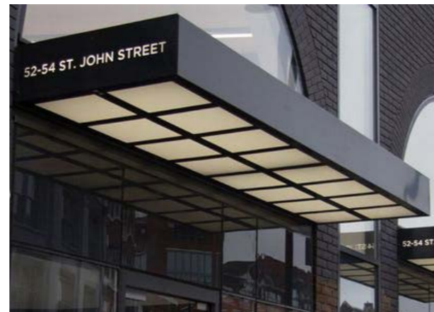
Fig.362 Simple canopy with illuminated underside
