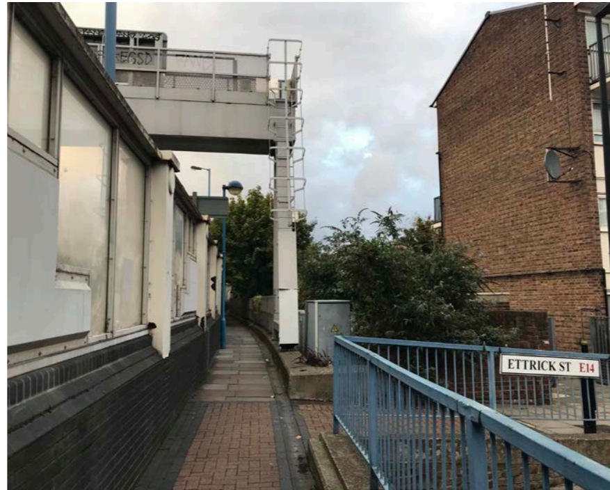
Fig.641 Narrow path to Bus stop with Gantry overhead
