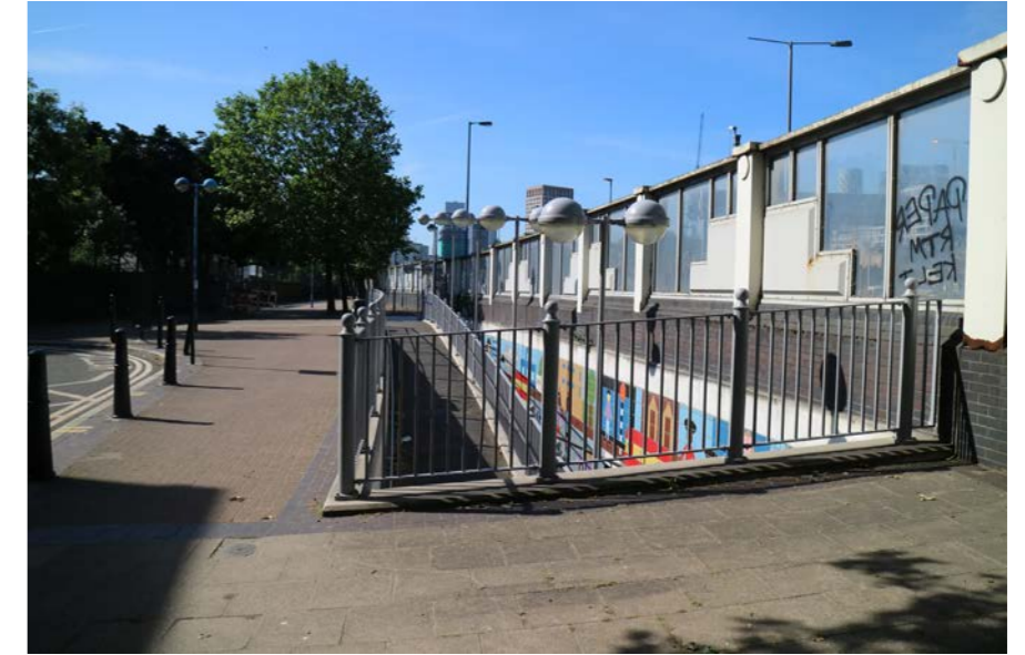
3 Fig.127 The pedestrian underpass at Dee Street
