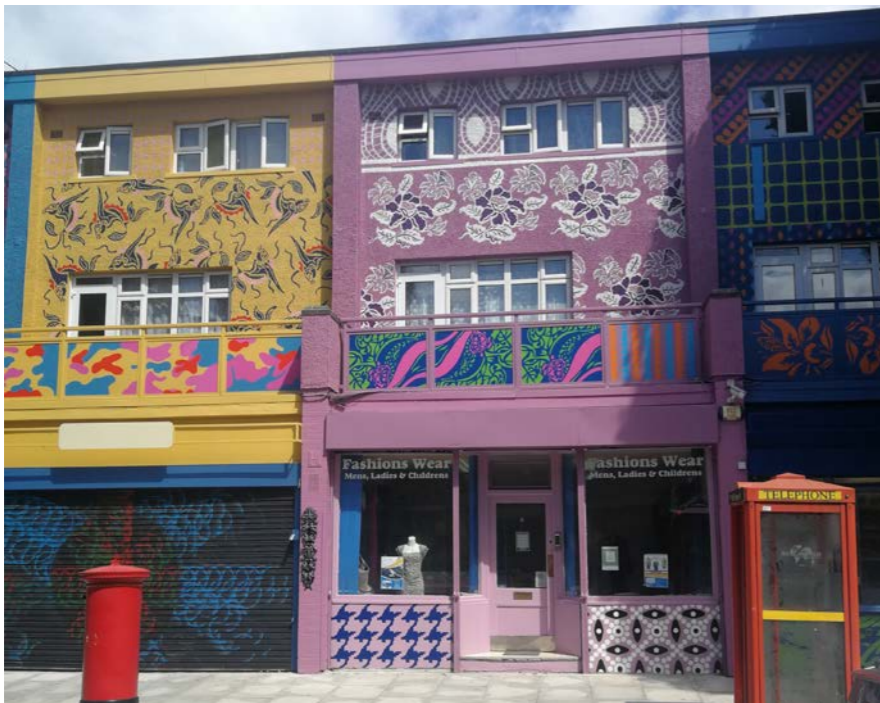
Fig.600 Existing colourful facade on Aberfeldy High Street
