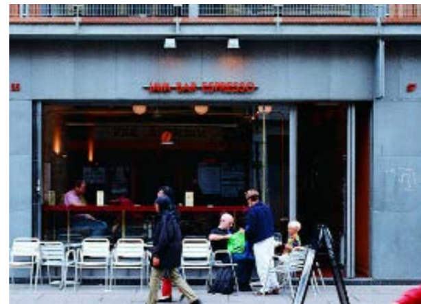
Fig.427 Concrete base with industrial aesthetic
