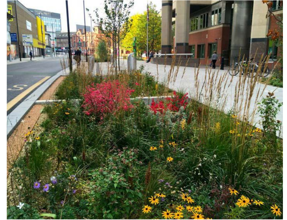
Fig.693 Rain gardens as part of a wider site surface water drainage strategy
