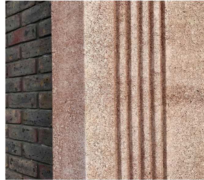
Fig.172 Textured panel with cast-in motif
