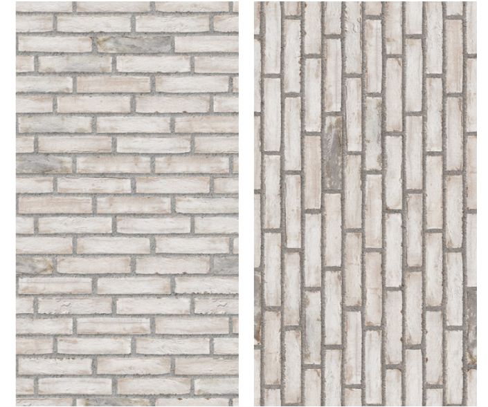
Fig.173 Pale brick with contrasting orientation and mortar colour
