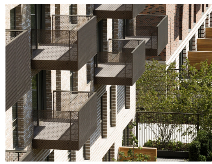
Fig.47 Projecting balconies - South Gardens, Elephant Park
