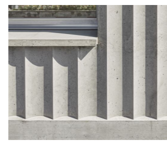
Fig.59 Textured concrete panel
