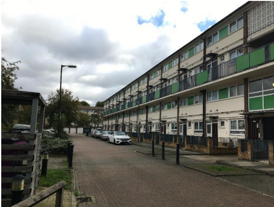
Figure 4.5 Typical hard surfaces
