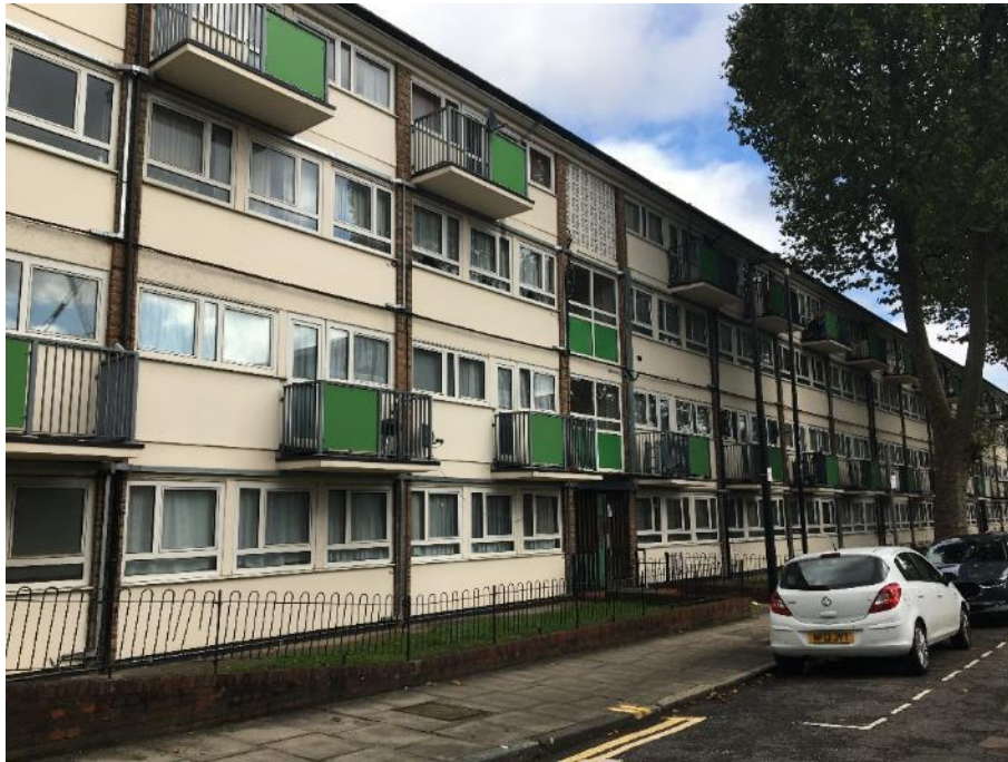
Figure 4.4 Residential flats in the main body of the site
