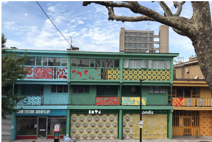
Figure 3-5 Building Exterior – Frontage
