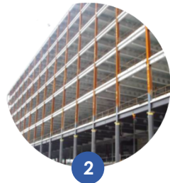
STEEL FRAME With profile concrete deck
