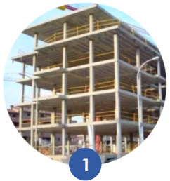
CONCRETE FRAME In-situ with flat slabs
