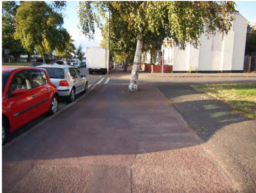
Figure 3.5 – Tree located in the footway
