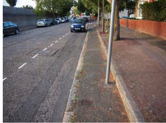
Figure 3.6 – Footway at difference levels
