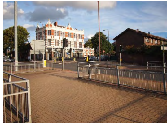
Figure 5.3 – Staggered pedestrian island
