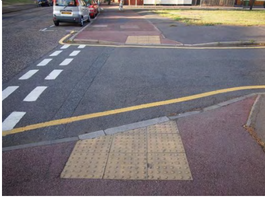
Figure 3.3 - Dropped kerbs and tactile paving
