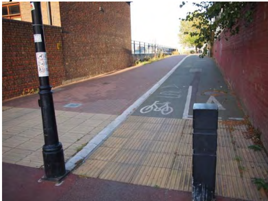
Figure 2.3 – Segregated footpath / cycle lane
