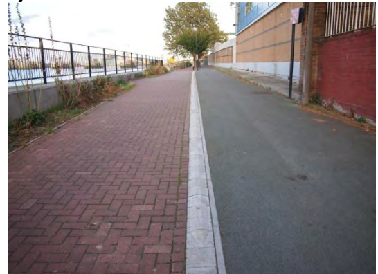
Figure 2.4 – Segregated footpath / cycle lane
