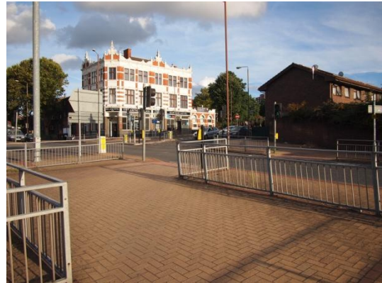
Figure 5.3 – Staggered pedestrian island
