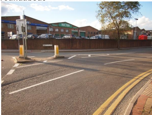
Figure 4.1 – Uncontrolled crossing at roundabout
