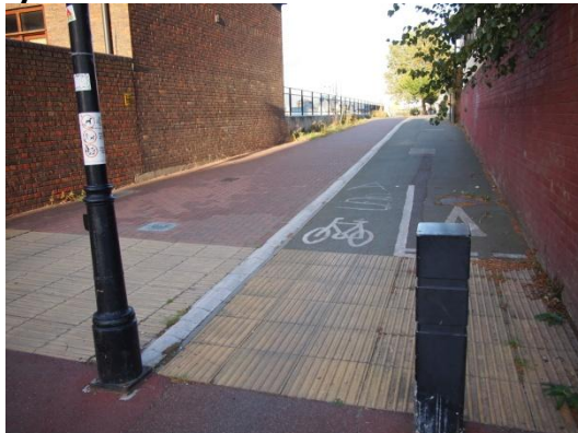
Figure 2.3 – Segregated footpath / cycle lane
