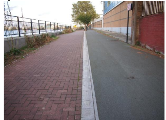
Figure 2.4 – Segregated footpath / cycle lane
