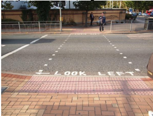
Figure 5.2 – Woolwich Road western arm pedestrian crossing
