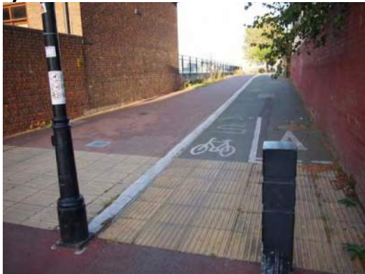
Figure 2.3 – Segregated footpath / cycle lane
