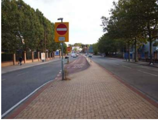
Figure 4.3 – Segregated bus lane
