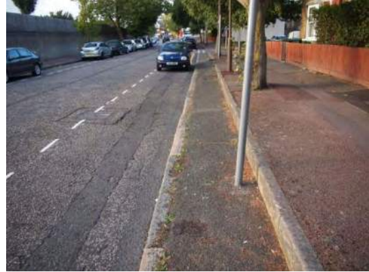
Figure 3.6 – Footway at difference levels
