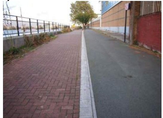
Figure 2.4 – Segregated footpath / cycle lane
