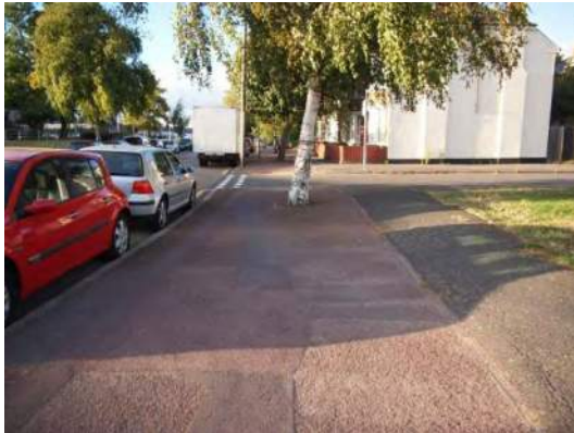
Figure 3.5 – Tree located in the footway
