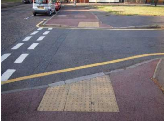
Figure 3.3 - Dropped kerbs and tactile paving
