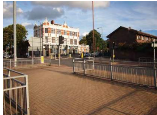
Figure 5.3 – Staggered pedestrian island
