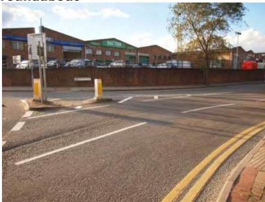
Figure 4.1 – Uncontrolled crossing at roundabout
