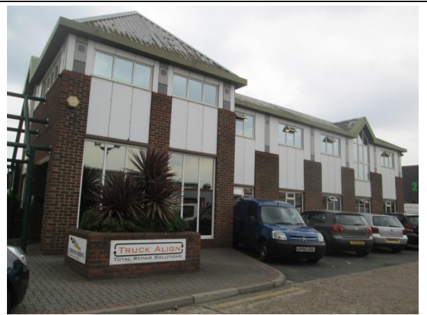
Unit to the north of the site
