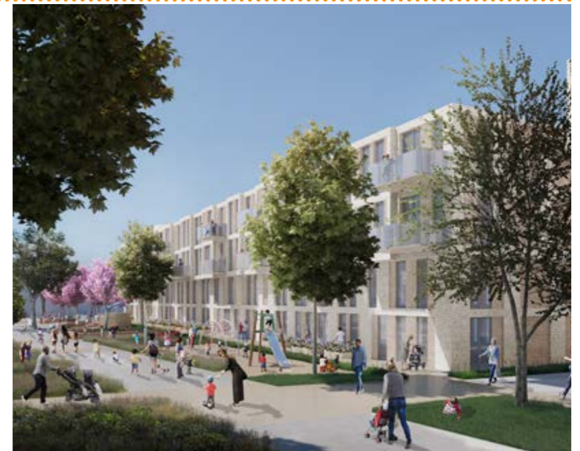
Playstreet -building H - 2 floors removed
