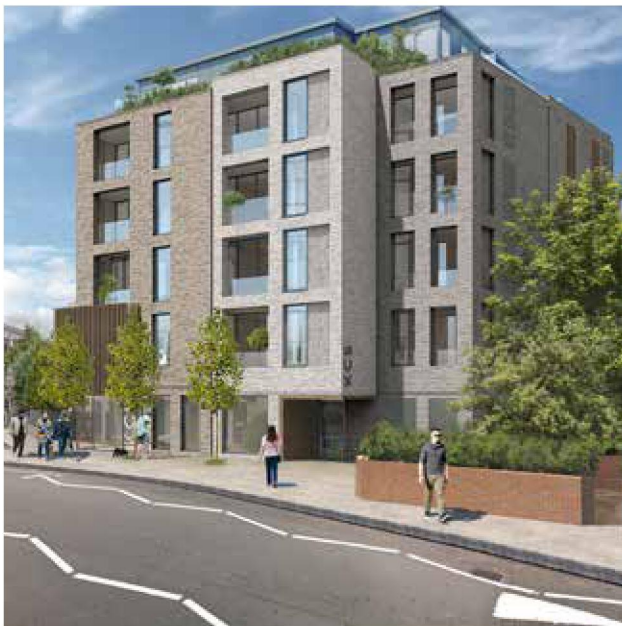
Kingston Community School, Coombe Road Consented: new primary school, sports hall, 19 new homes
