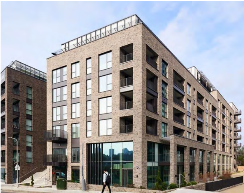
Legacy Wharf, Newham (5 – 8 storeys)
