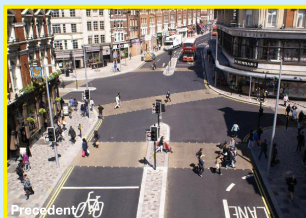
Precedent ^ St Johns Hill, Clapham Junction: creating a high street which works for multiple transport modes
