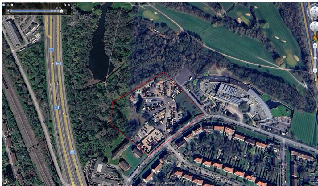
Image 1; The Google Earth satellite image shows the approximate site boundary in red. The image shows that the large majority of the site is urban and hardstanding and a small area is suitable for reptiles. The area to the north shows green spacer and widespread suitable habitat within proximity of the site (GoogleEarth, 2026).
