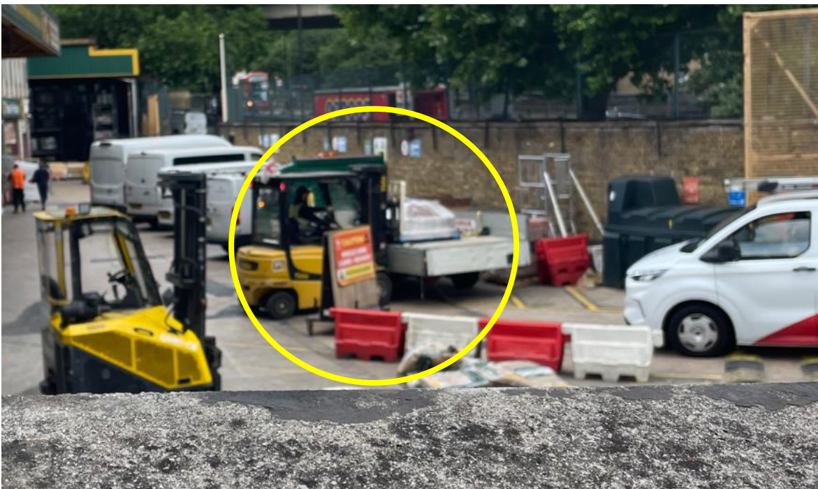
Figure 1 – Travis Perkins flatbed van – forklift truck loading materials with stopboard deployed
