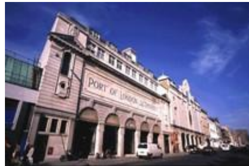
Figure 1 – Citigen Energy Centre (Photo courtesy of E.On UK Ltd)
