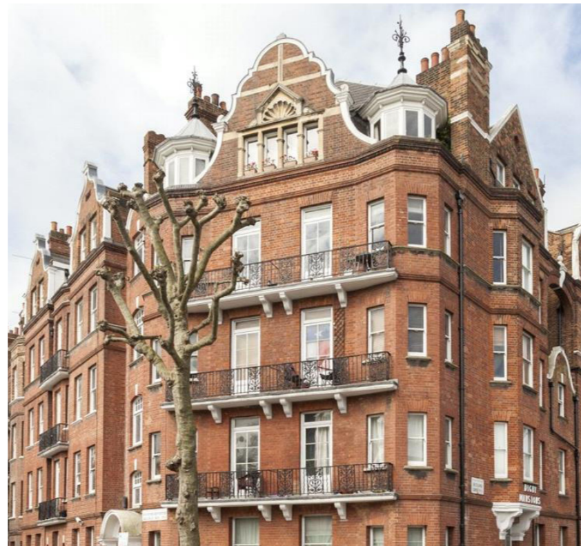
Digby Mansions (street facing facade)
