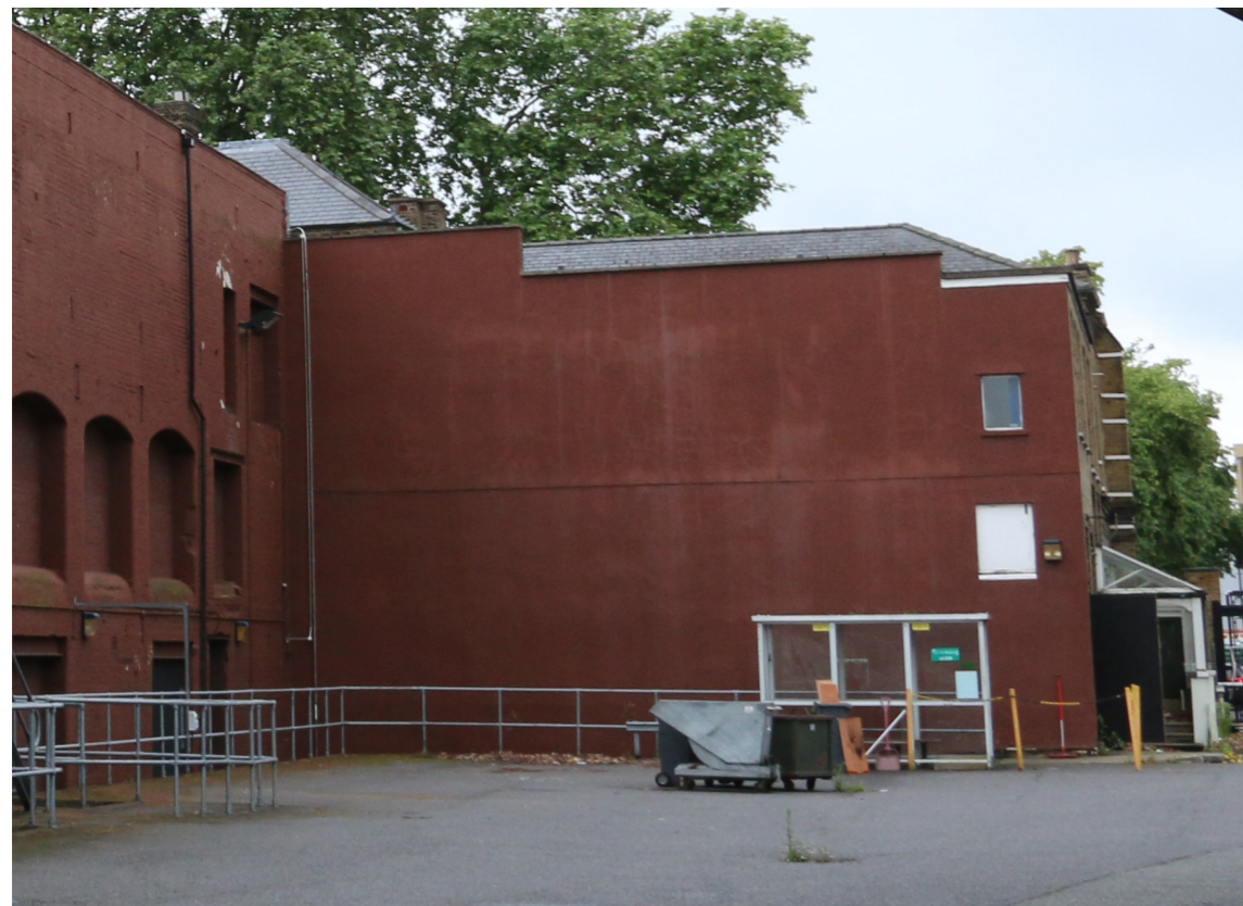
Existing east elevation of former hotel building
