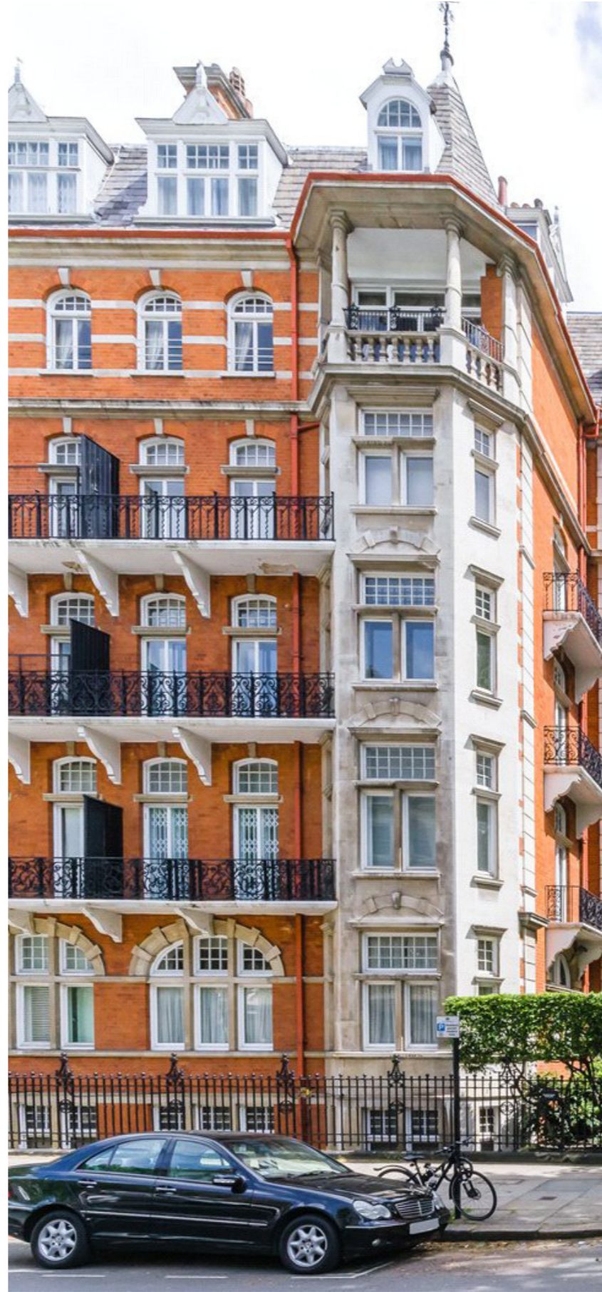
Alexandra Court - exsample of vertical hierarchy within balustrade design
