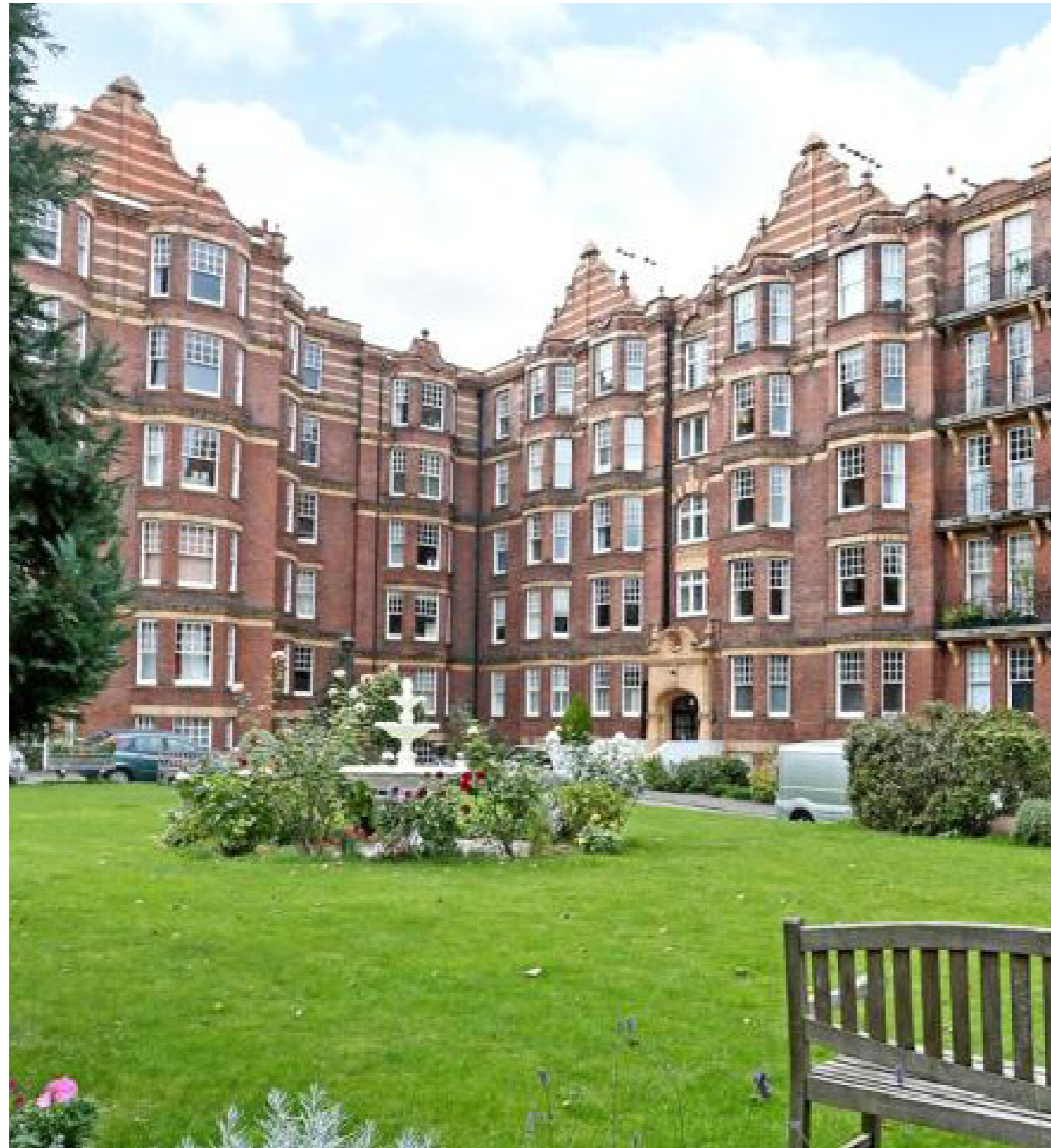
Exterior photograph of Kenilworth Court
