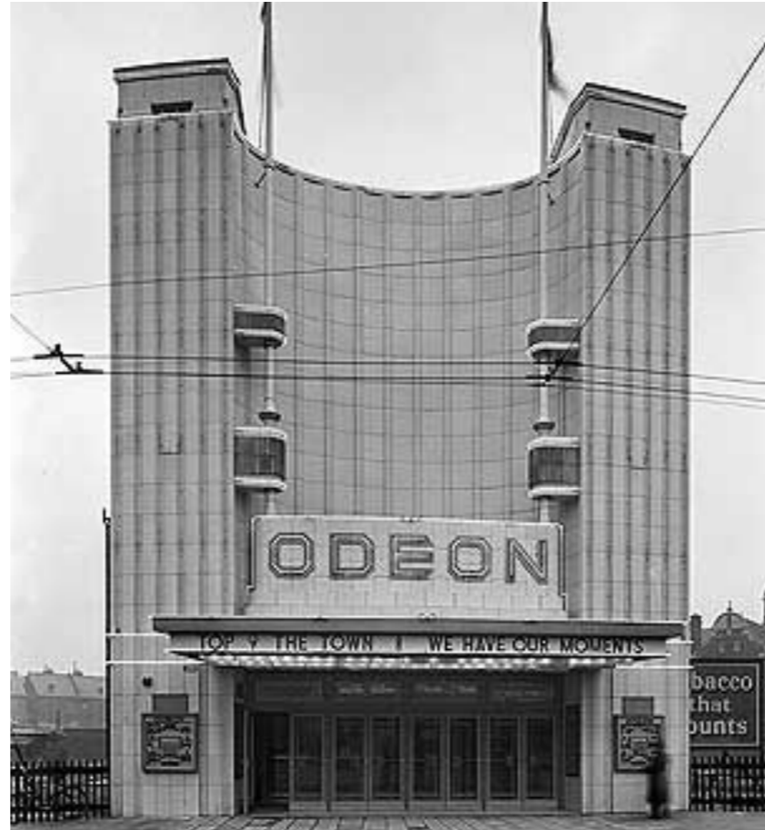
Example of decorative masonry - Odeon cinema, Southsea, Portsmouth
