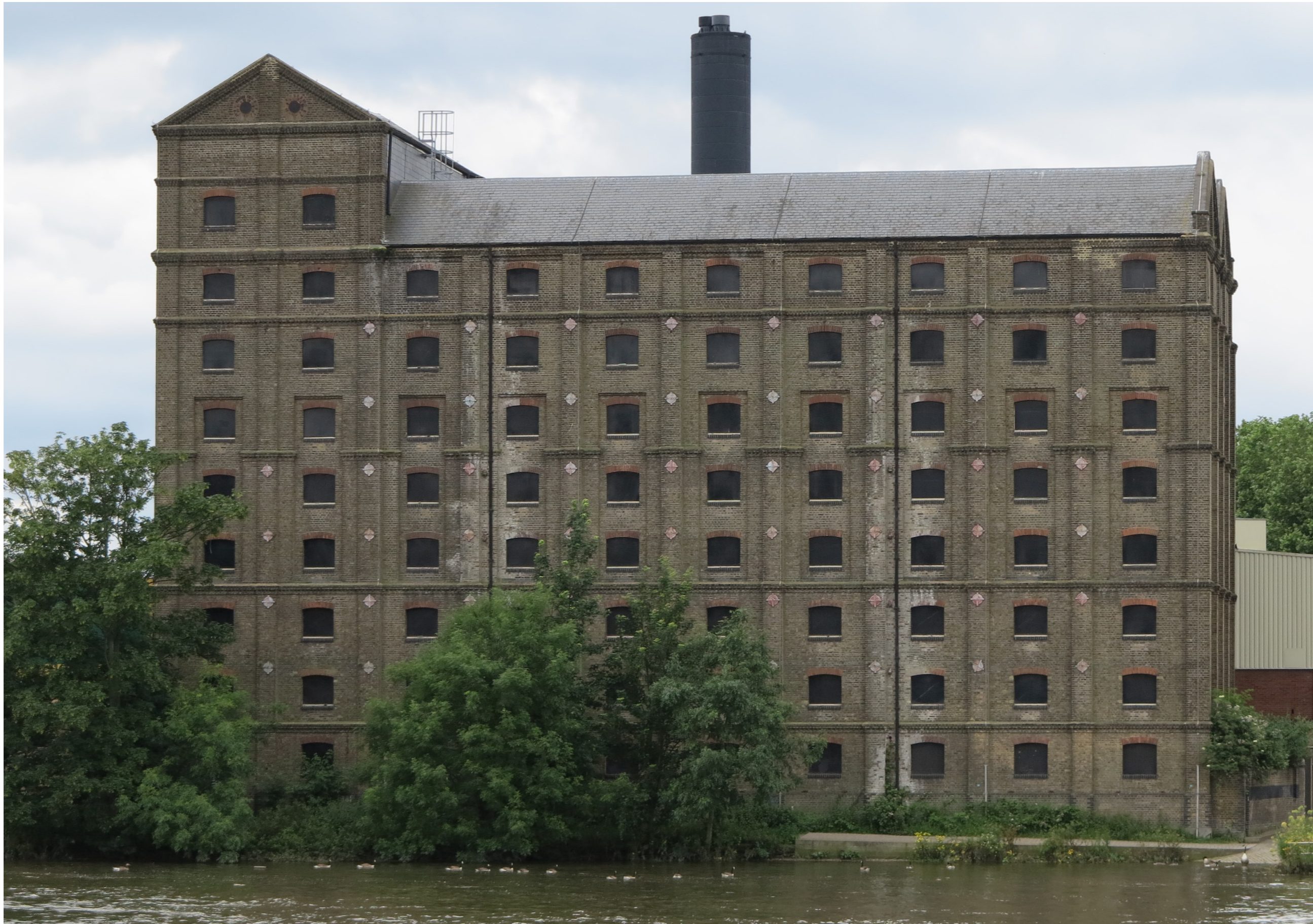
Photograph of existing Maltings building
