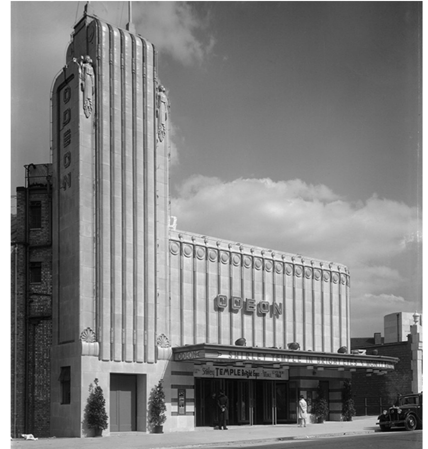
Example of decorative masonry - Odeon cinema, Chingford Mount
