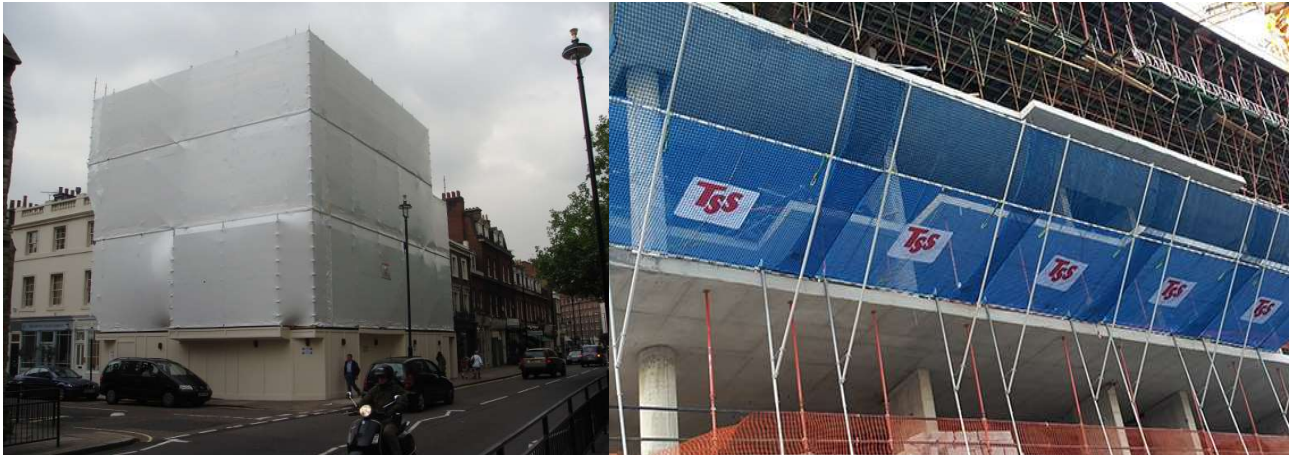
Figures 11 & 12: Full Building Scaffolding and Safety Fans
