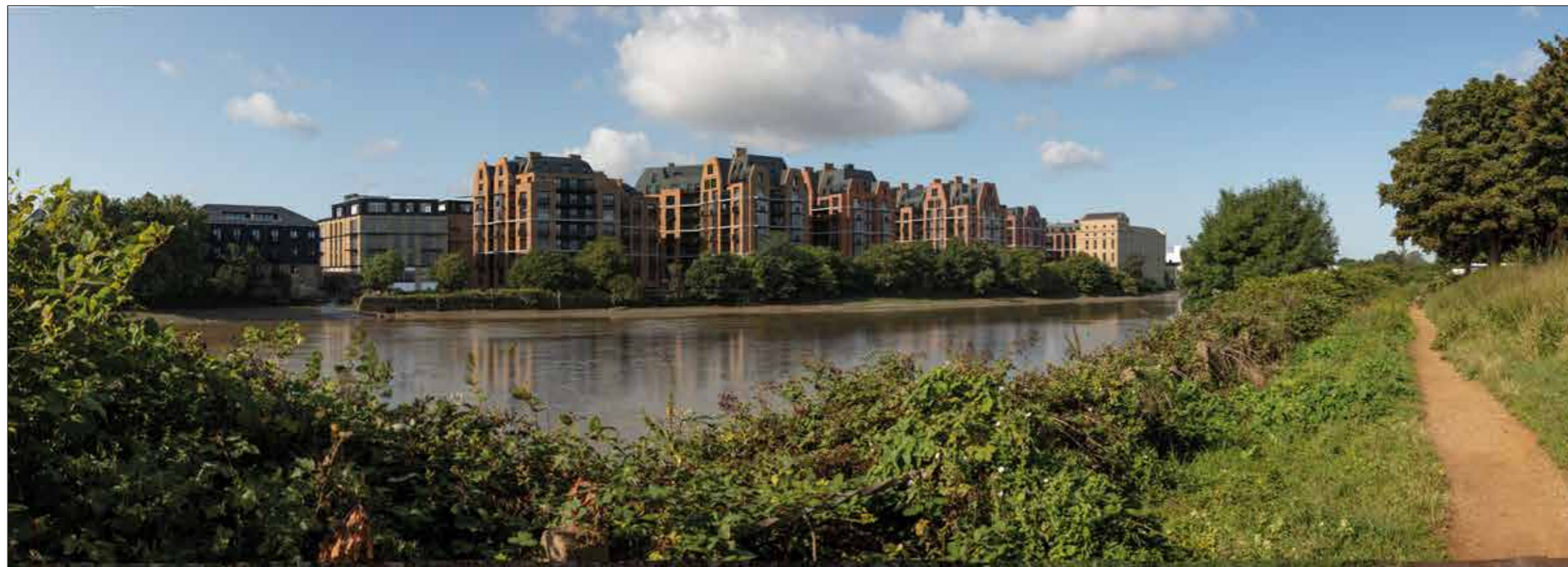
Viewpoint 6: Proposed view from the Thames Path (north) adjacent to the car parking area on Dan Mason Drive, looking southwest across the River Thames towards the Stag Brewery component of the Site.
