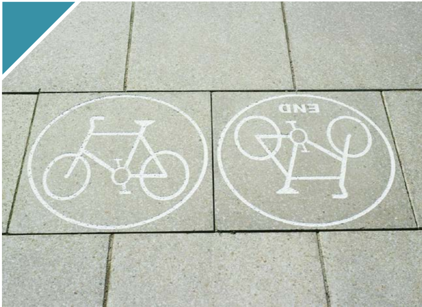
Artificial Stone Flag Paving
