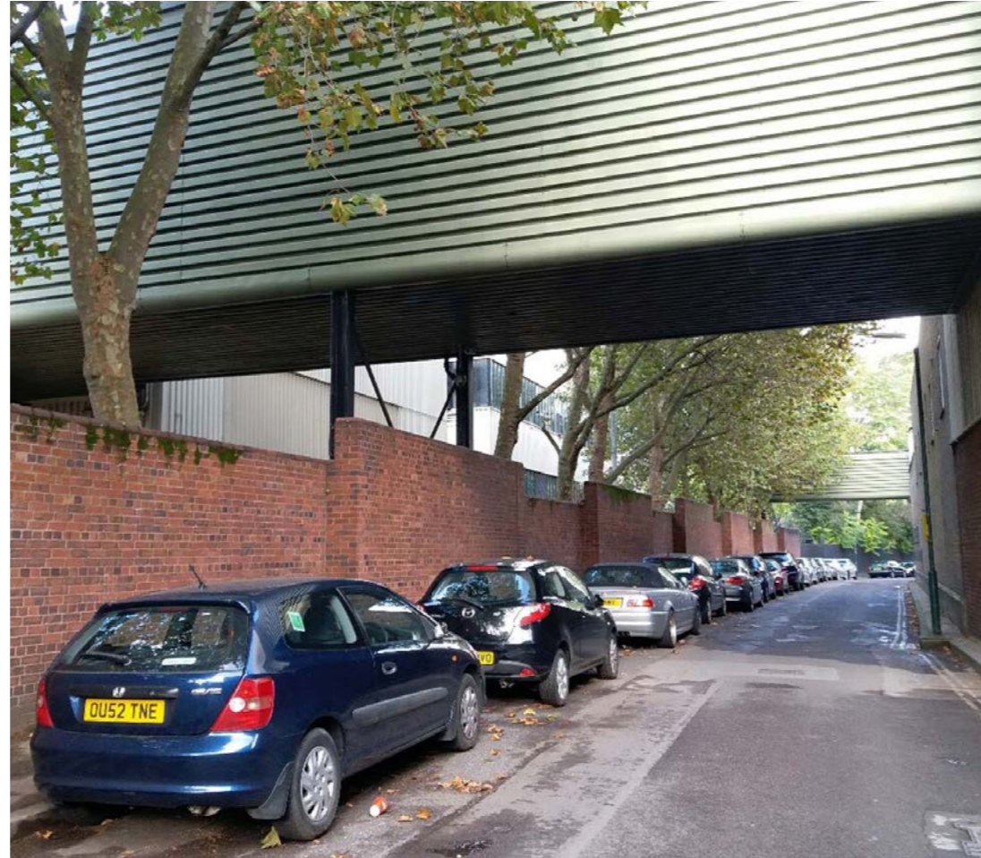
SHIP LANE (SITE SURROUND)
