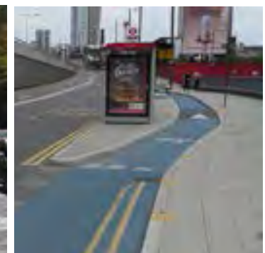
Bus stop bypass, Stratford High Street, London
