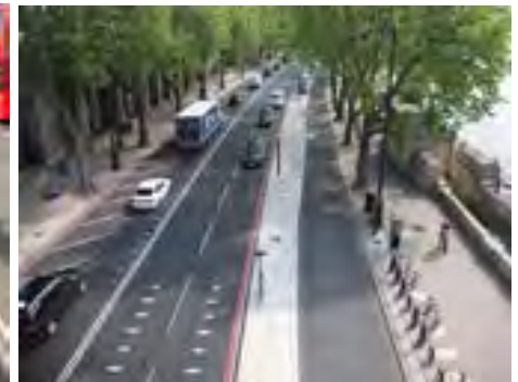
Full separation, East West Cycle Superhighway
