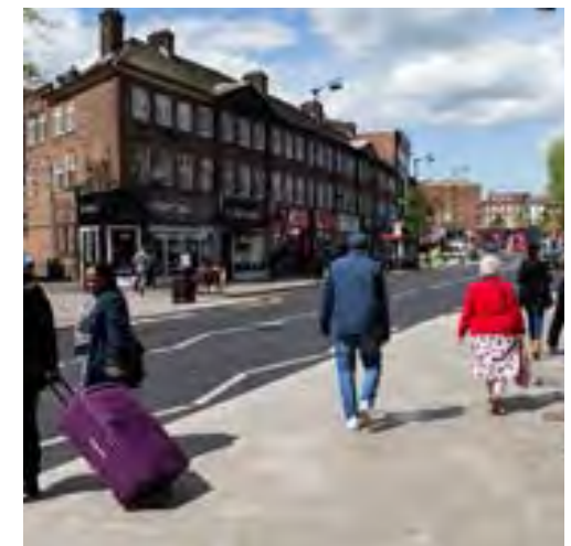
Top: Inset bays, Wood Green Above: resurfacing and de-cluttering, Wood Green
