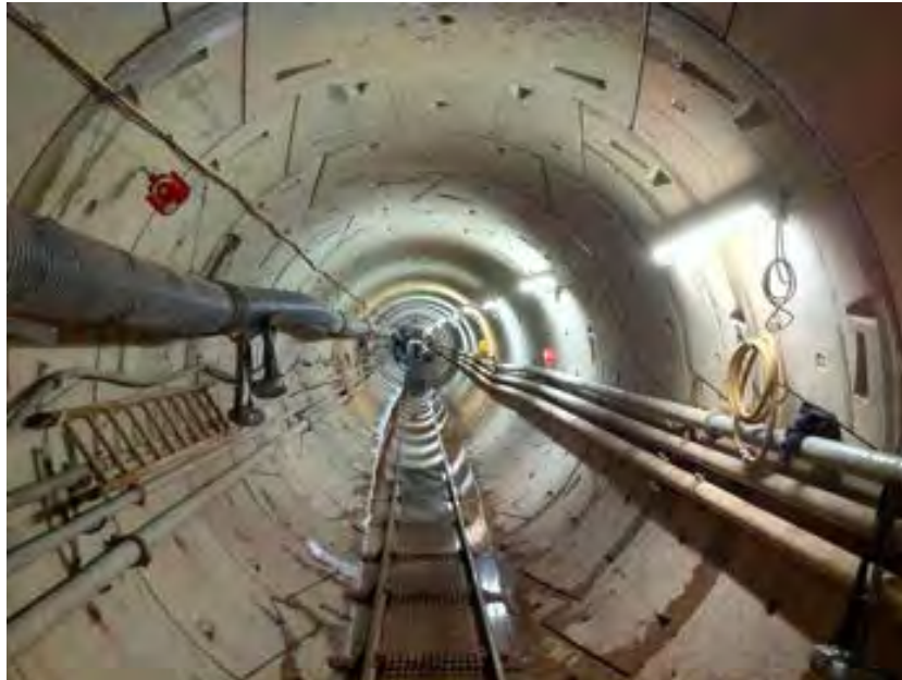
Image of a service subway
