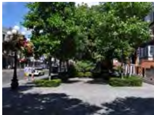
Permeable paving, Islington Town Hall
