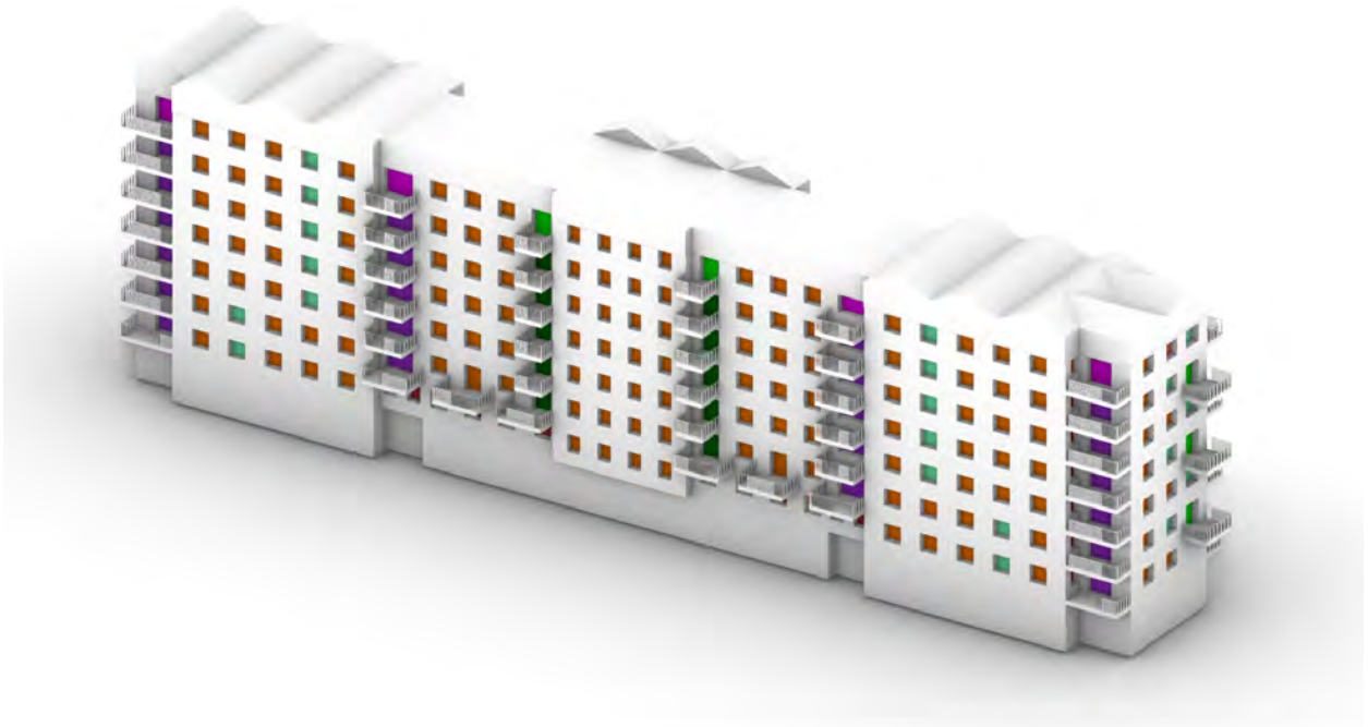
Fig. 04: North-east view - Block_H1-H2
