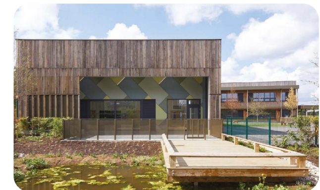
FIG 1.27 Sustainable design of school buildings; Hackbridge School. Image credit: studiostagg; available at Resilient London - NLA
