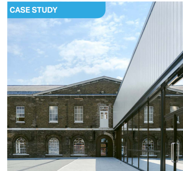
FIG 4.37 Royal Arsenal, Woolwich: Grade II and Grade II* buildings have been transformed into flexible space for performance, events, training and education. Image credit: divisare
