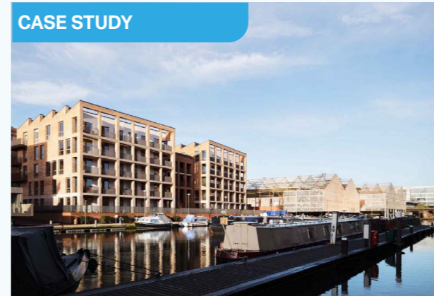
FIG 3.53 Brentford Lock West is a development providing views to water and high-quality public realm establishing the canal-side as a desirable place to live and visit. Image credit: Mae architects
