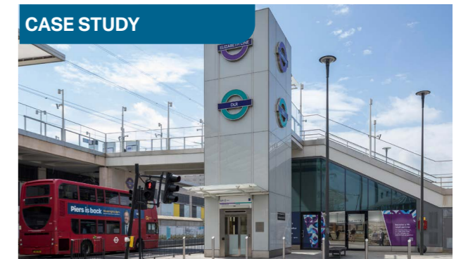
FIG 5.13 Custom House station has recently been rebuilt and a new mezzanine level constructed to improve access to ExCeL London as well as provide the DLR interchange with the Elizabeth Line
