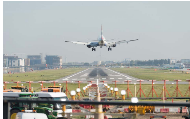
FIG 1.9 London City Airport. Image credits: Tian Khee Siong
