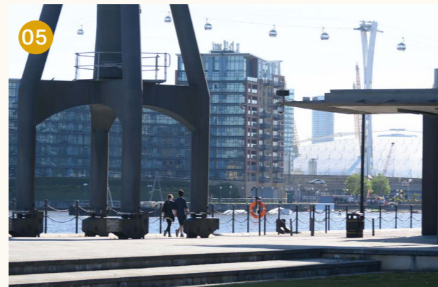
FIG 3.101 Listed dock structures. Image credit: Tian Khee Siong
