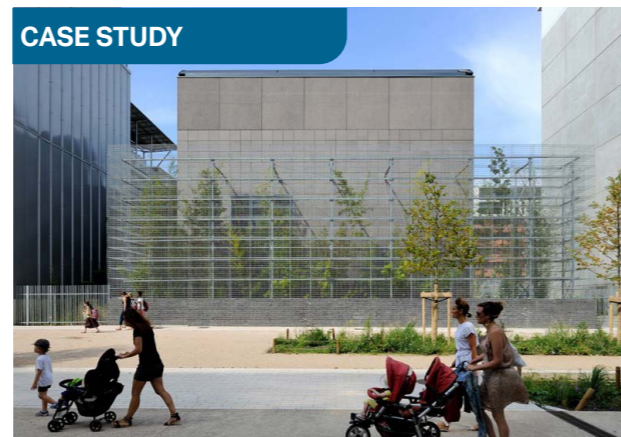
CASE STUDY FIG 6.6 Primary Substation, Lyon, France. Image credit: Studio Erick Salliet
