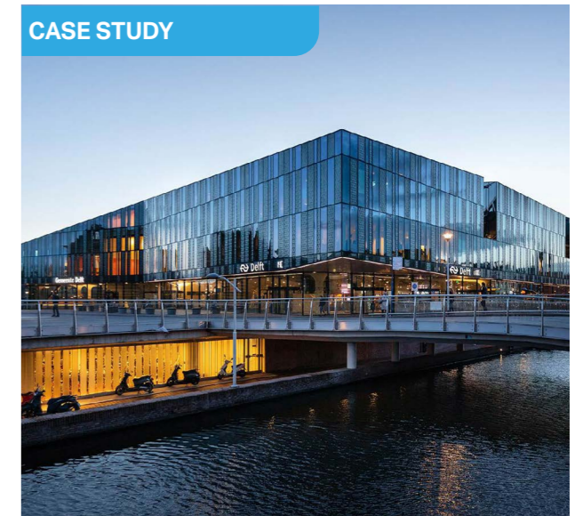
FIG 4.48 In Delft, The Netherlands the new train station created a new piece of city unlocking the water, enabling walking and cycling routes, attracting a range of town centre uses and steering new development. Image credit: Mecanoo
