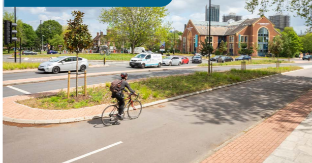
FIG 5.14 Improved bus and cycle corridor along Jamaica Road in Bermondsey. A new eastbound bus gate on the Jamaica Road approach to Rotherhithe roundabout gives buses priority and easier access into Lower Road. The scheme includes new and improved street layout, landscaping and segregated cycle lanes.
