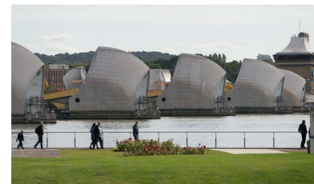
FIG 1.21 Existing connections. Image credit: Tian Khee Siong
