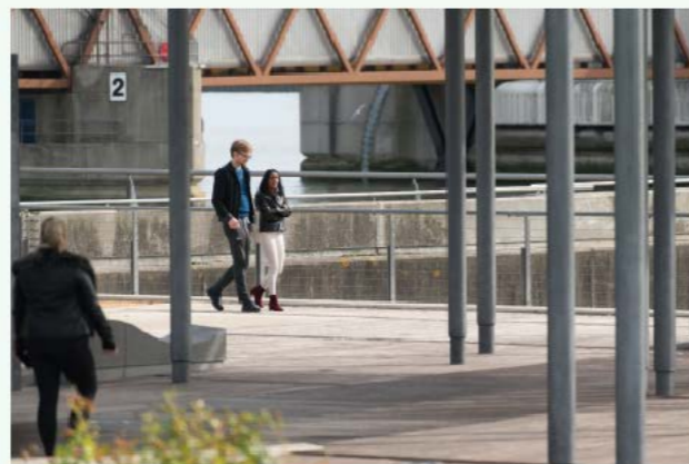
FIG 3.68 Thames Barrier . Image credits: Tian Khee Siong
