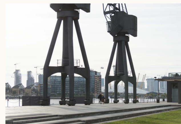
FIG 3.7 Listed cranes at Victoria dock. Image credit: Tian Khee Siong
