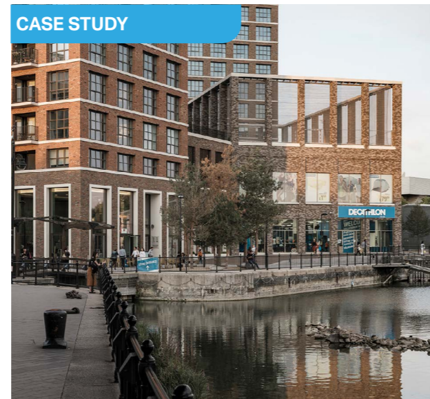
FIG 4.46 Canada Water, London. Area transformed into a new mixed-use town centre that has the intimacy and animation of a traditional high street. Image credit: Tim Crocker
