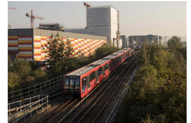
FIG 1.4 Major transport infrastructure investment. Image credit: Sam Bush
