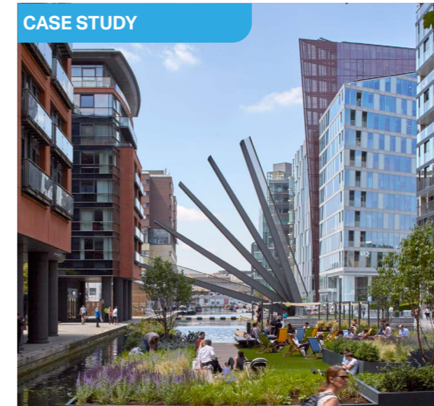
FIG 4.24 Merchant Square, London. High-quality development with public realm and open space along water canals. Image credit: Divisare
