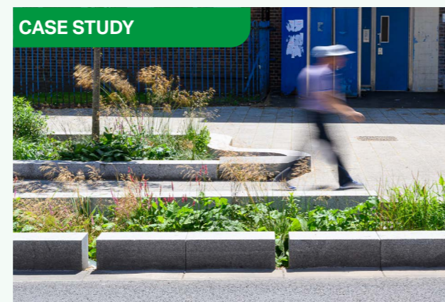
FIG 3.64 Vegetated rain-gardens form part of new road improvements in White Hart Lane, Tottenham. Image credit: Robert Bray Associates
