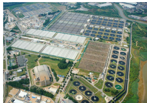
FIG 6.3 Beckton Sewage treatment
