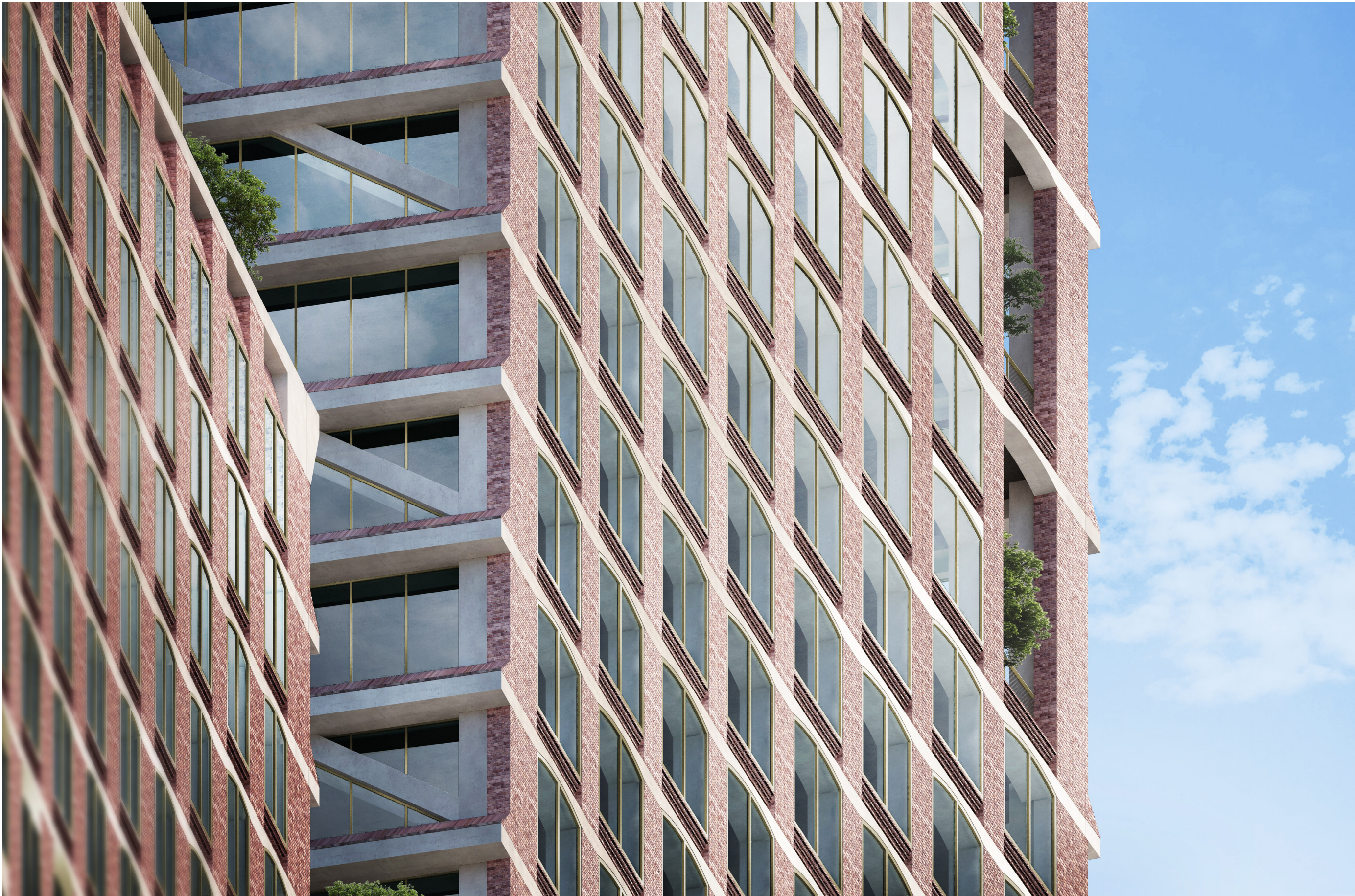
Fig. 4.8.5.3 North Façade detail view
