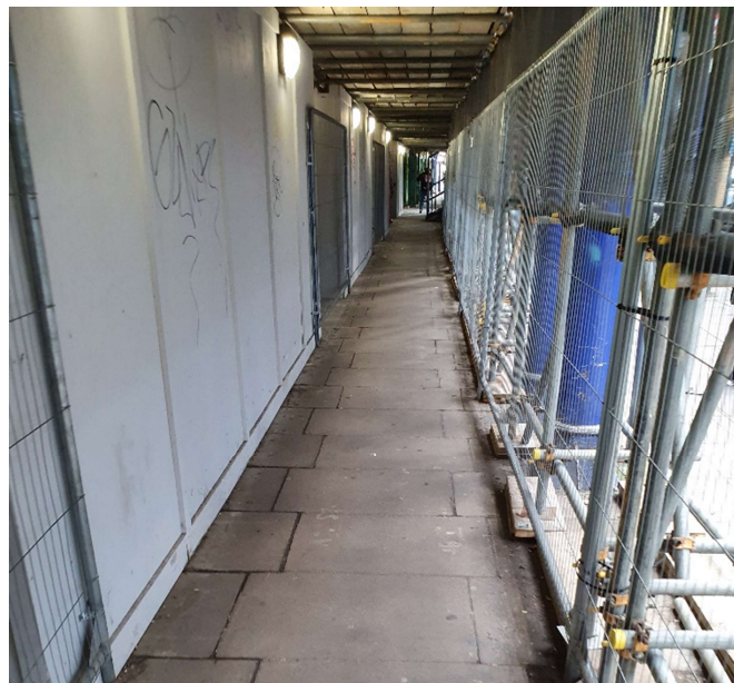
Photograph 4: Footway along Atlantic Road northern side.
