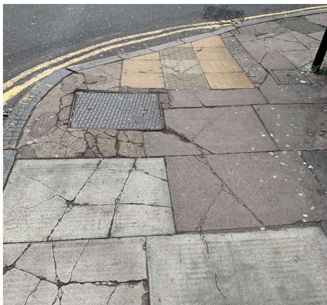
Photograph 3: Footway along Atlantic Road southern side.
