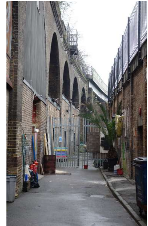
Fig. 2.12.2.6 View from street looking west
