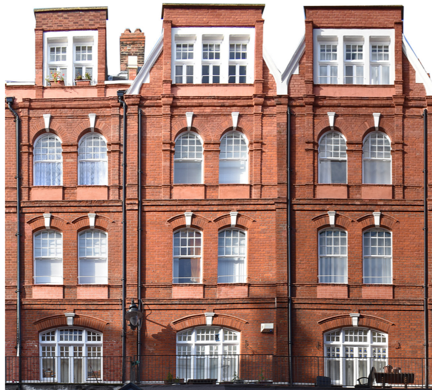
Fig. 3.6.3.4 Building facade on Electric Avenue
