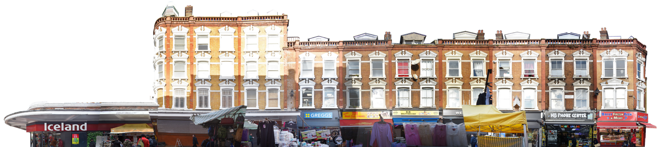
Fig. 3.6.5.2 Building facades on Electric Avenue south west
