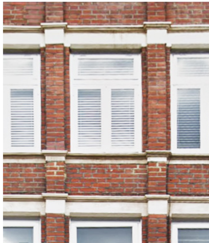
Fig. 3.6.4.3 Brick & Concrete detailing of building facade on Coldharbour Lane
