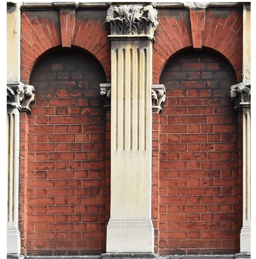
Fig. 3.6.4.5 Brick & Concrete detailing of building facade on Coldharbour Lane
