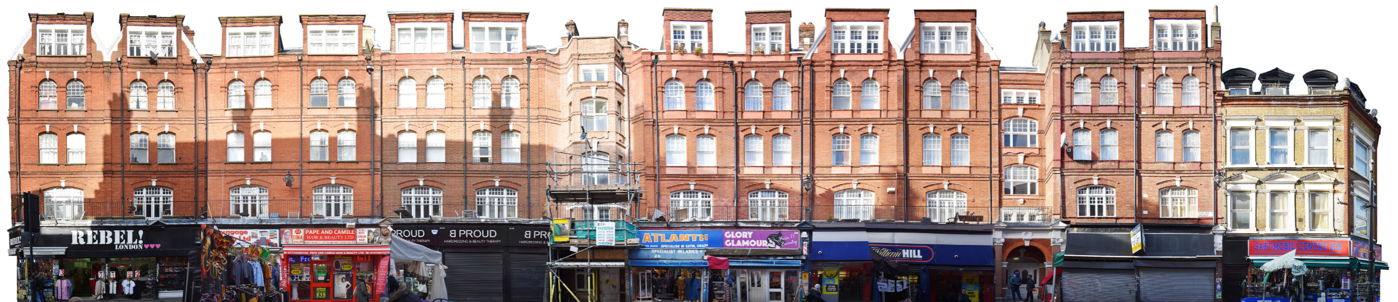
Fig. 3.6.5.4 Building facades on Electric Avenue north west
