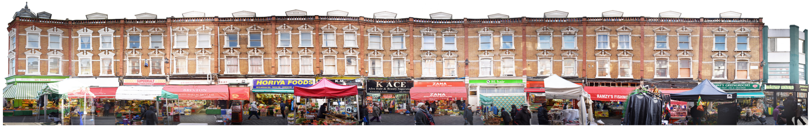
Fig. 3.6.5.1 Building facade on Electric Avenue north east
