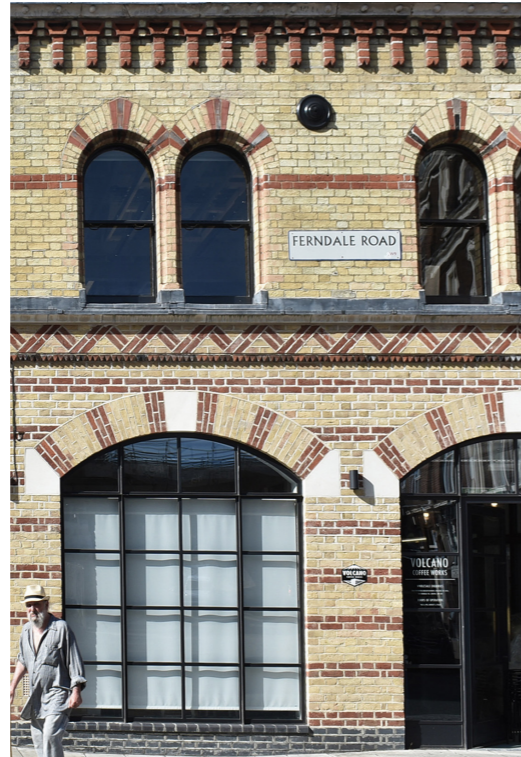
Fig. 3.6.3.1 Building facade on Ferndale Road
