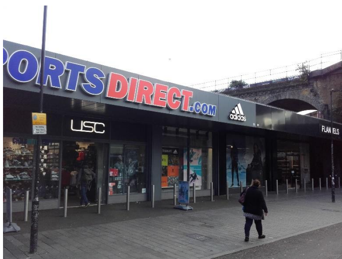
Photograph 3 Western aspect of building B1, fronting onto Pope's Road.
