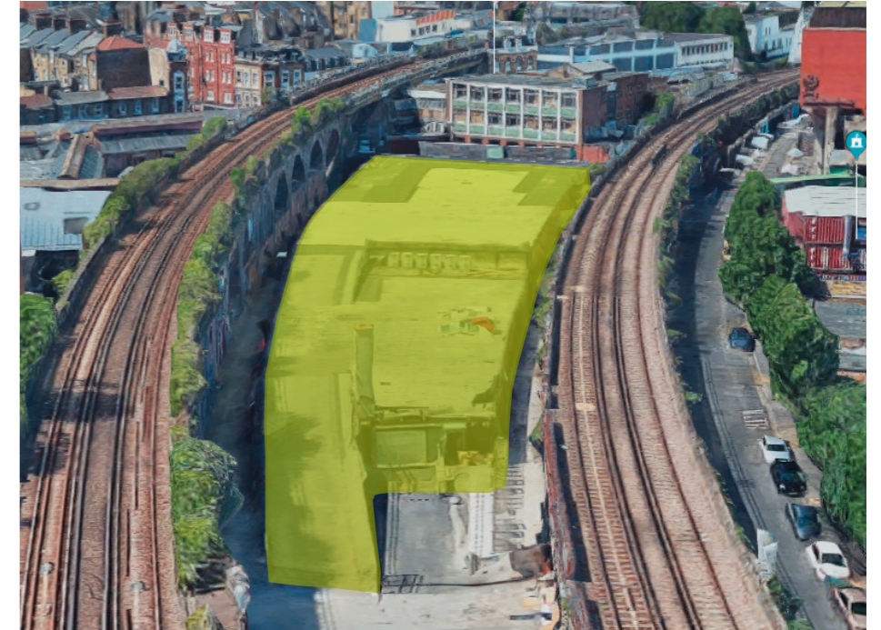
Figure 3.11 East to west view of existing structure
