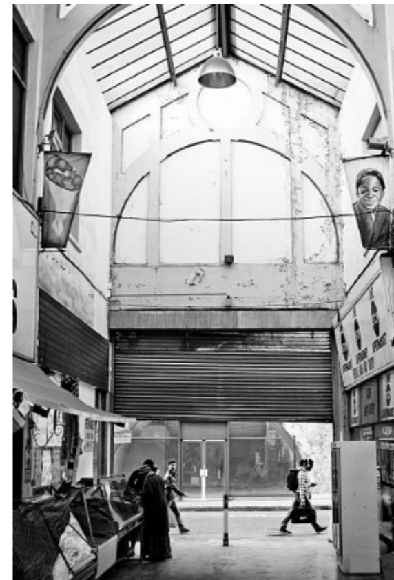
Fig. 2.4.4.4 Market Row Interior at east entrance towards Atlantic Road, c 1970
