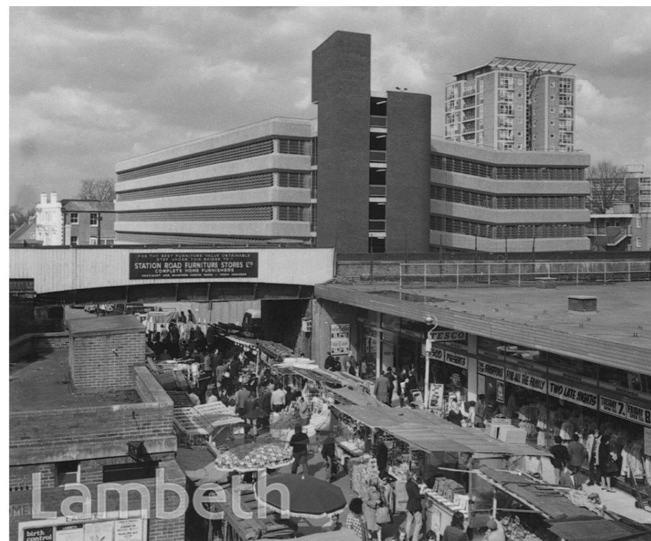
Fig. 2.4.5.3 Pope's Road looking north with Tesco on current application site, street market and multi-storey car park, 1974
