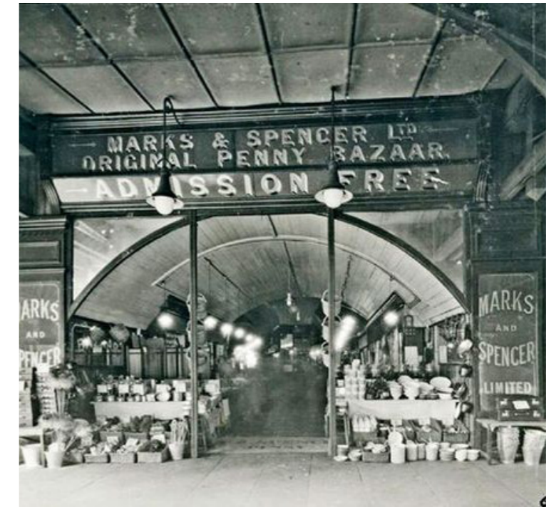
Fig. 2.4.2.2 Original Marks and Spencer located under Brixton Railway Viaduct, 1920
