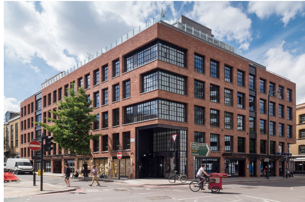
1.3.1.1 External view of The Curtain, Shoreditch, London
