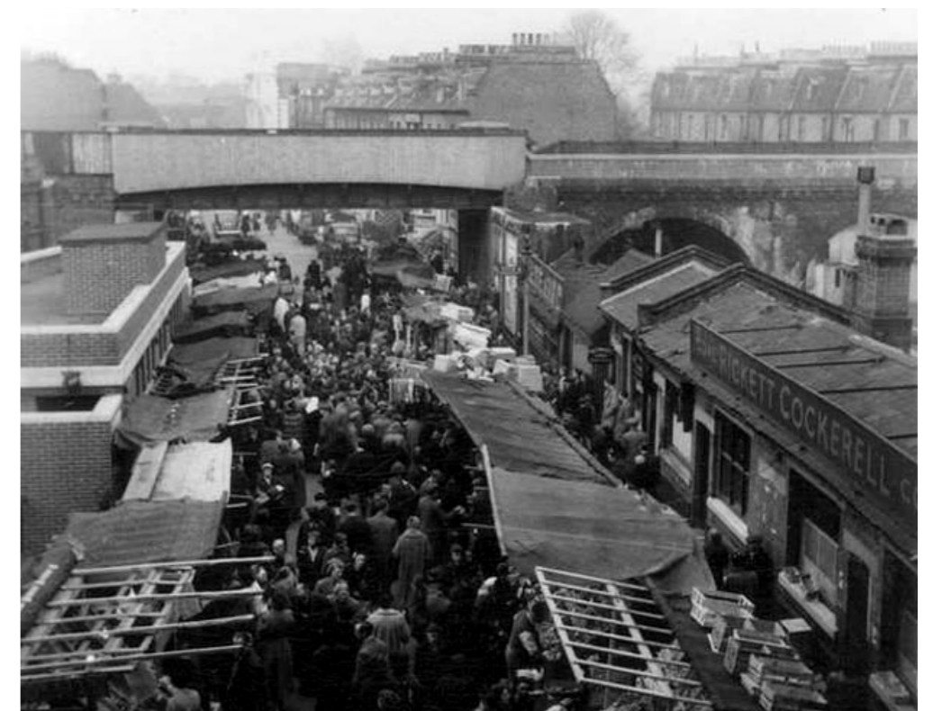
Fig. 2.4.5.4 Pope's Road looking north with street market, 1956
