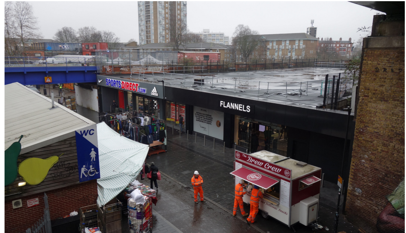
Fig. 2.1.1 Aerial view of Pope's Road looking north east
