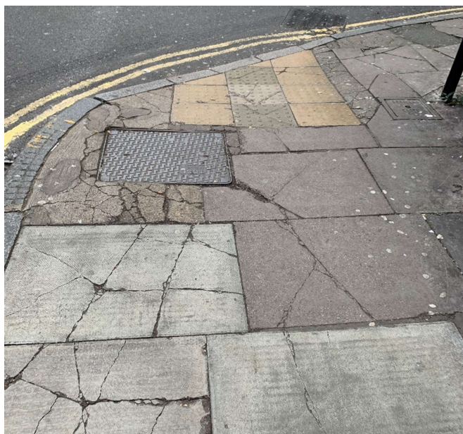
Photograph 3: Footway along Atlantic Road southern side.
