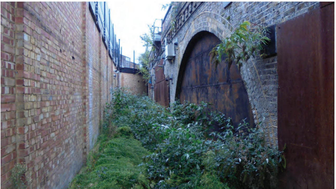
Plate 6: View of the north-west corner of the Site, facing west
