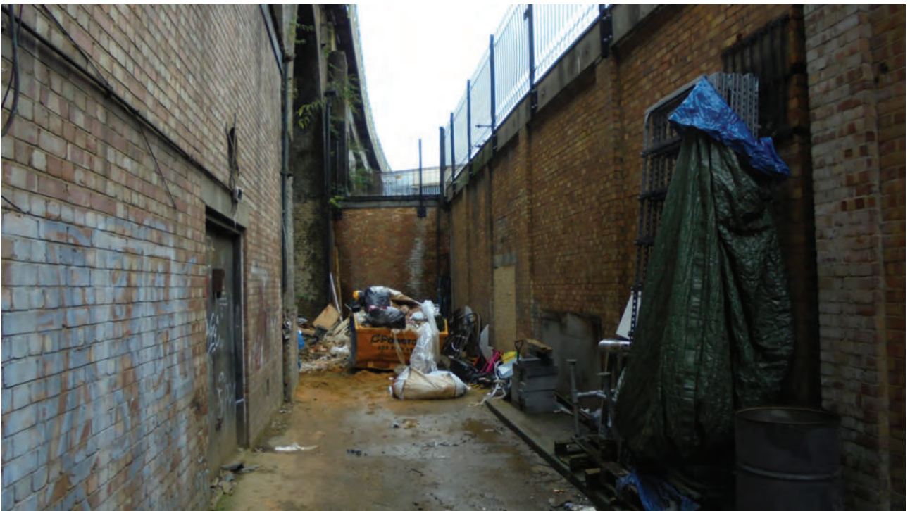
Plate 4: View of the south-west corner of the Site, facing west
