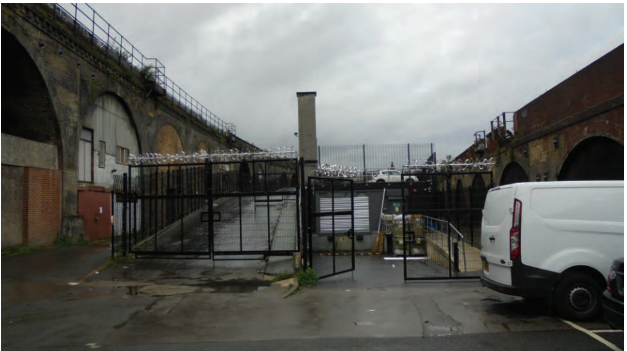
Plate 2: General view of the Site and the rear of the retail unit, facing west
