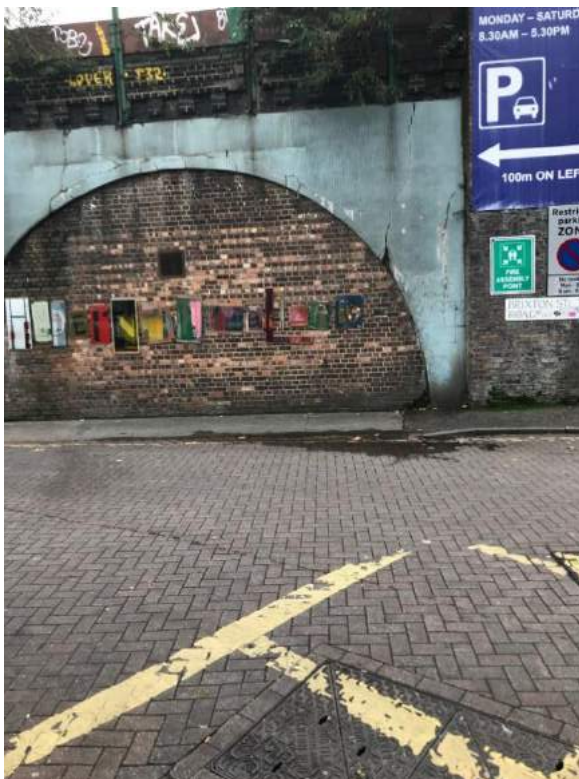
Photo 4: Onsite railway arch fronting Brixton Station Road, (Bricked with no access).
