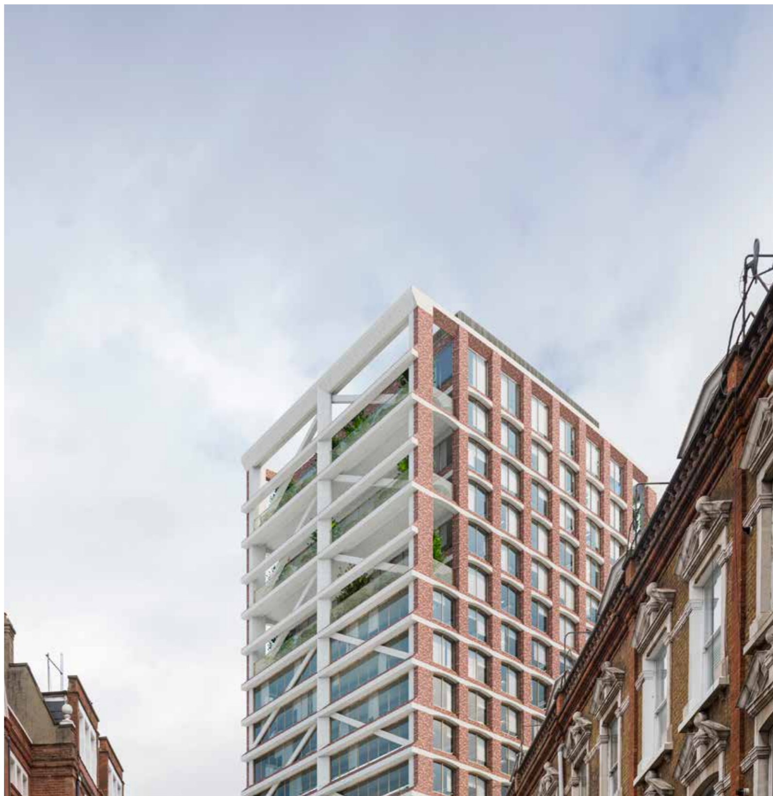
Fig. 2.2.1.2 September 2020 Planning Addendum south-west facade top part illustrative close up view
