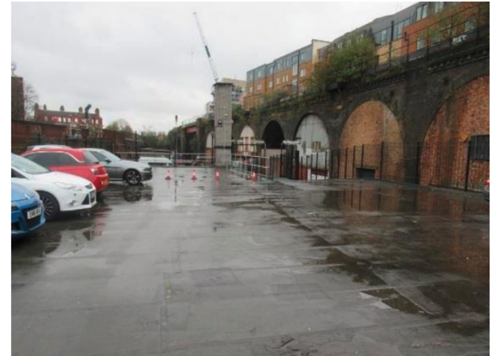
Figure 3.13 Car park located on roof
