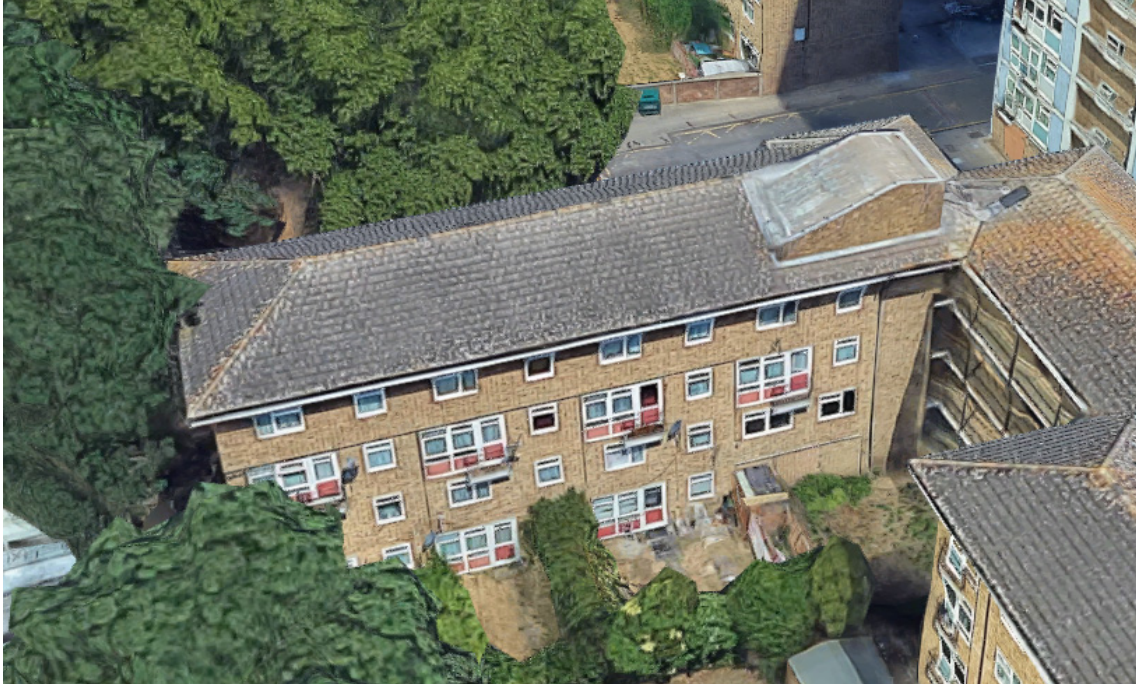
Figure 10: Image of Wincheap Court
