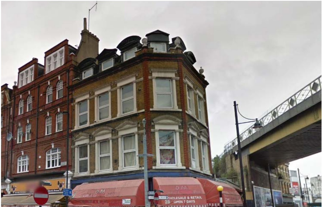
Figure 12: Image of 28 Atlantic Road
