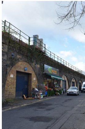
Existing facade of Brixton Station Road
