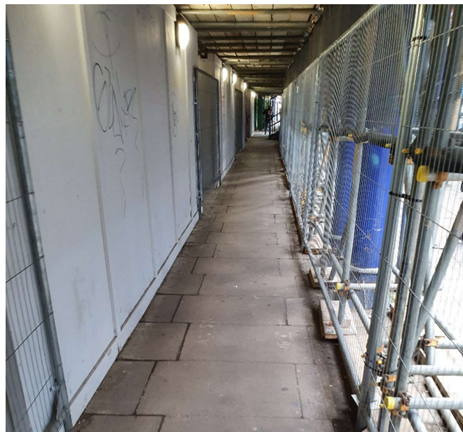
Photograph 4: Footway along Atlantic Road northern side.
