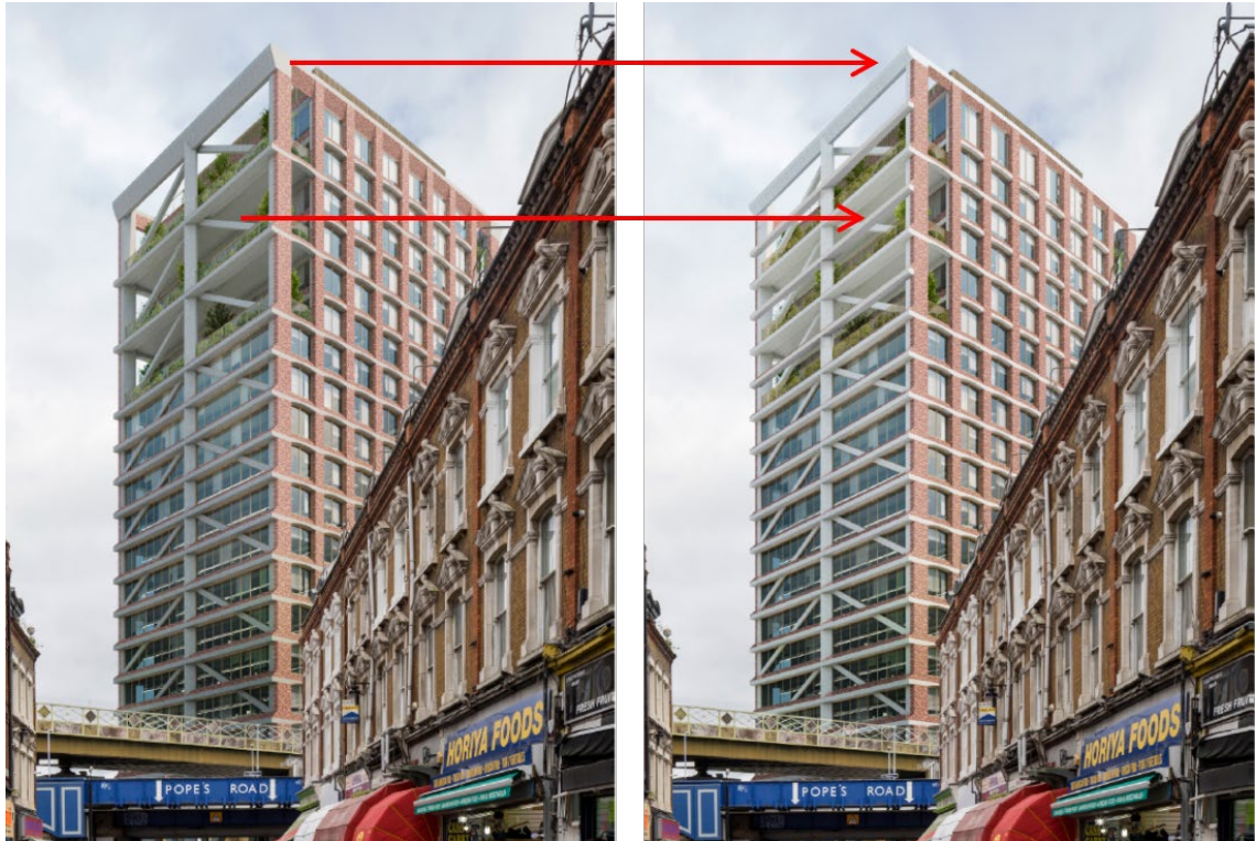
Figure 1: Proposed amendments to terrace levels and crown (left - as tested, right - proposed amendments)
