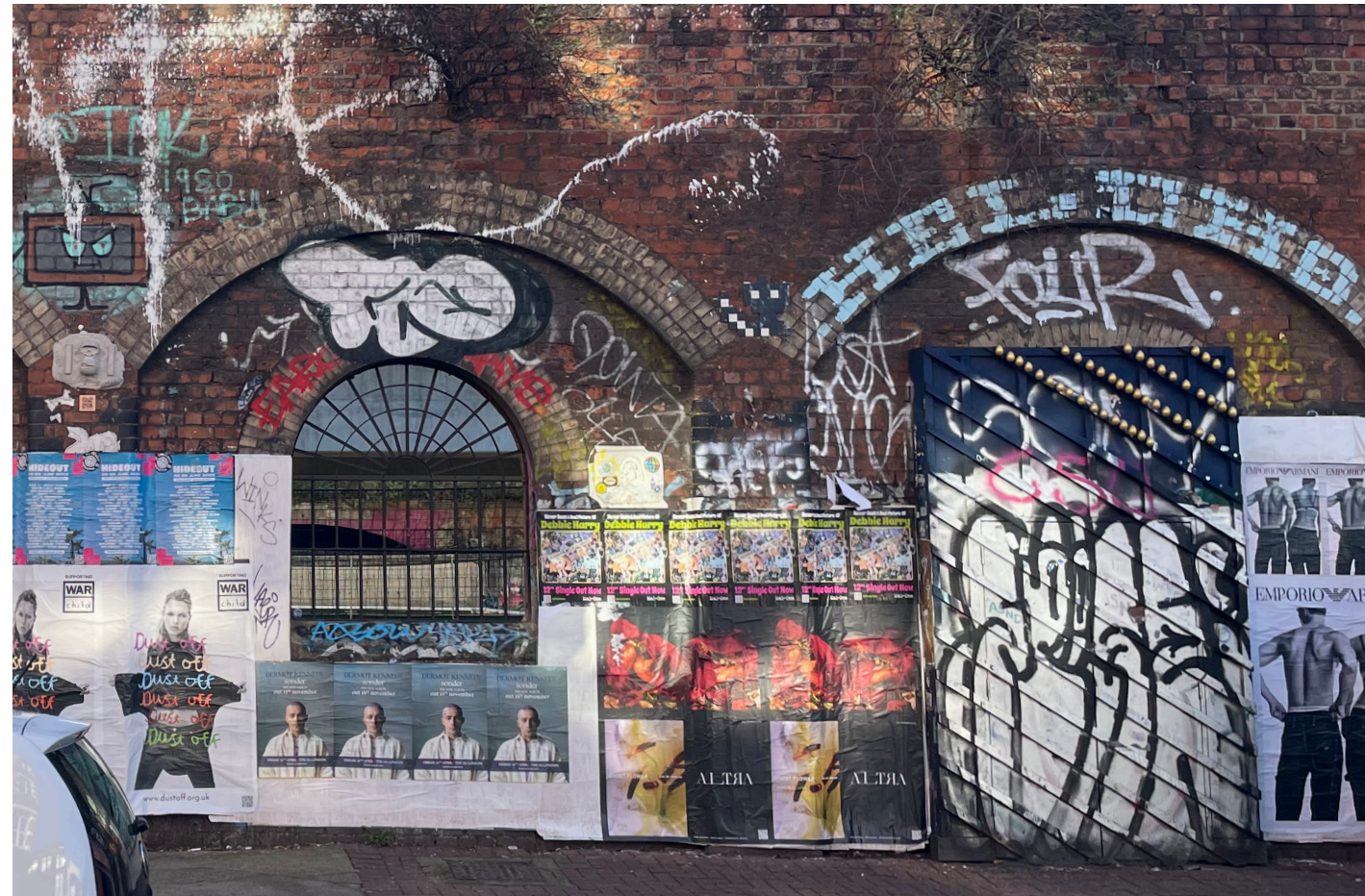
Existing arched wall
