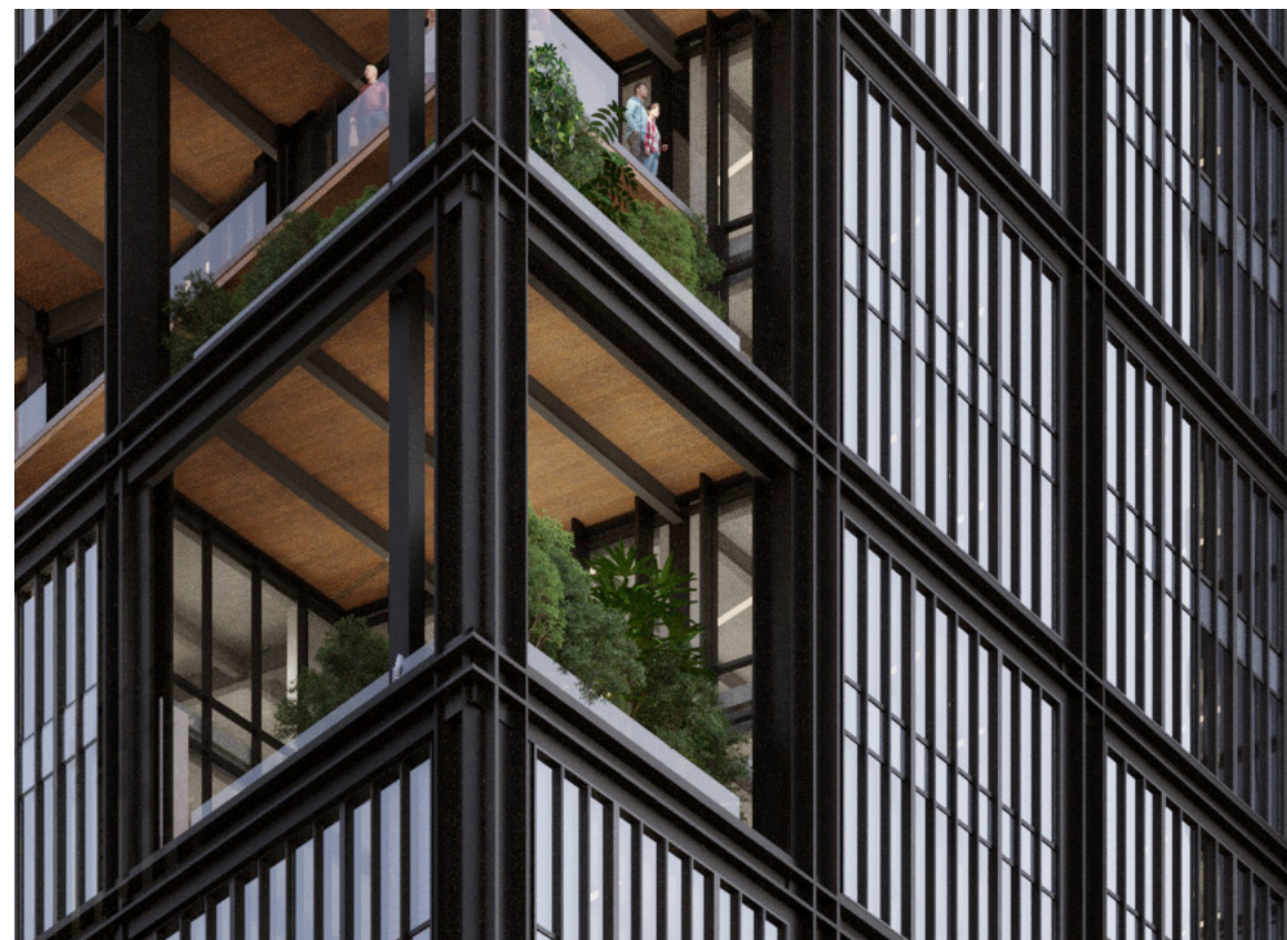
Lightweight steel frame upper floors
