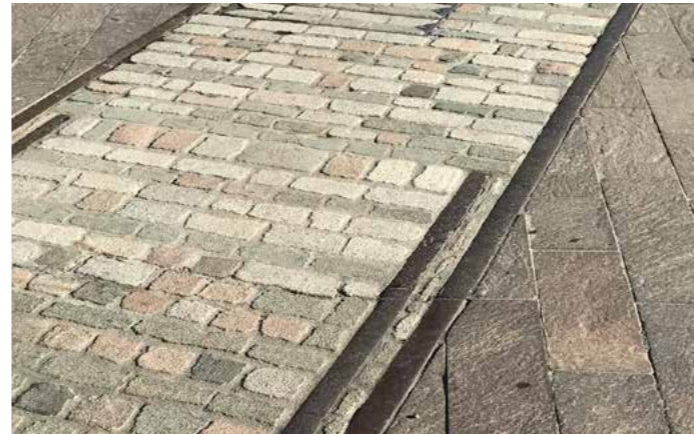
Reclaimed granite setts, flush historic rails, and porphyry paving at Granary Square, Kings Cross
