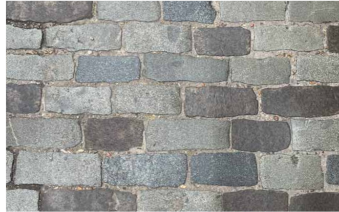
Existing granite setts, showing the variation in tone
