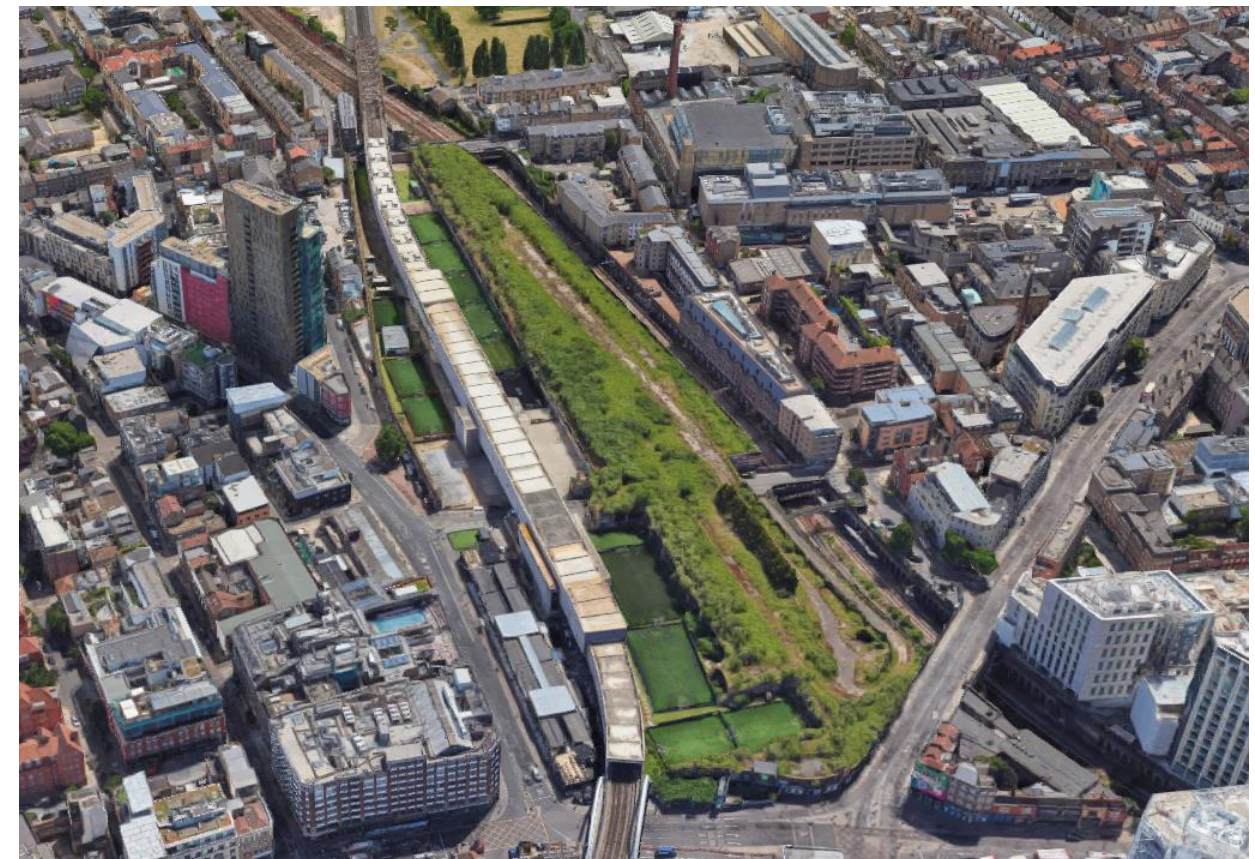
Figure 4 Aerial view of existing site
