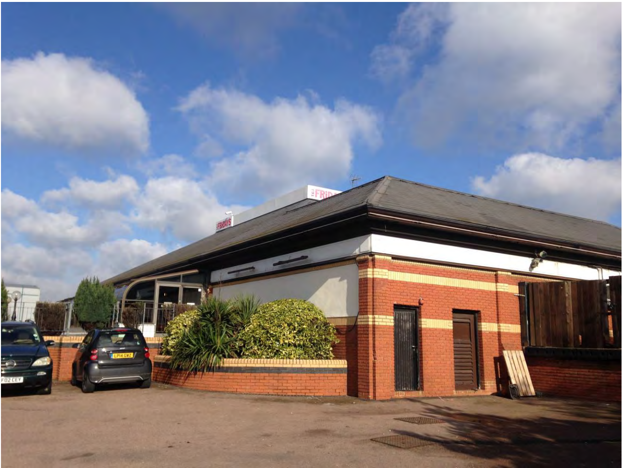
Figure 26: View east showing side elevation of TGI Fridays
