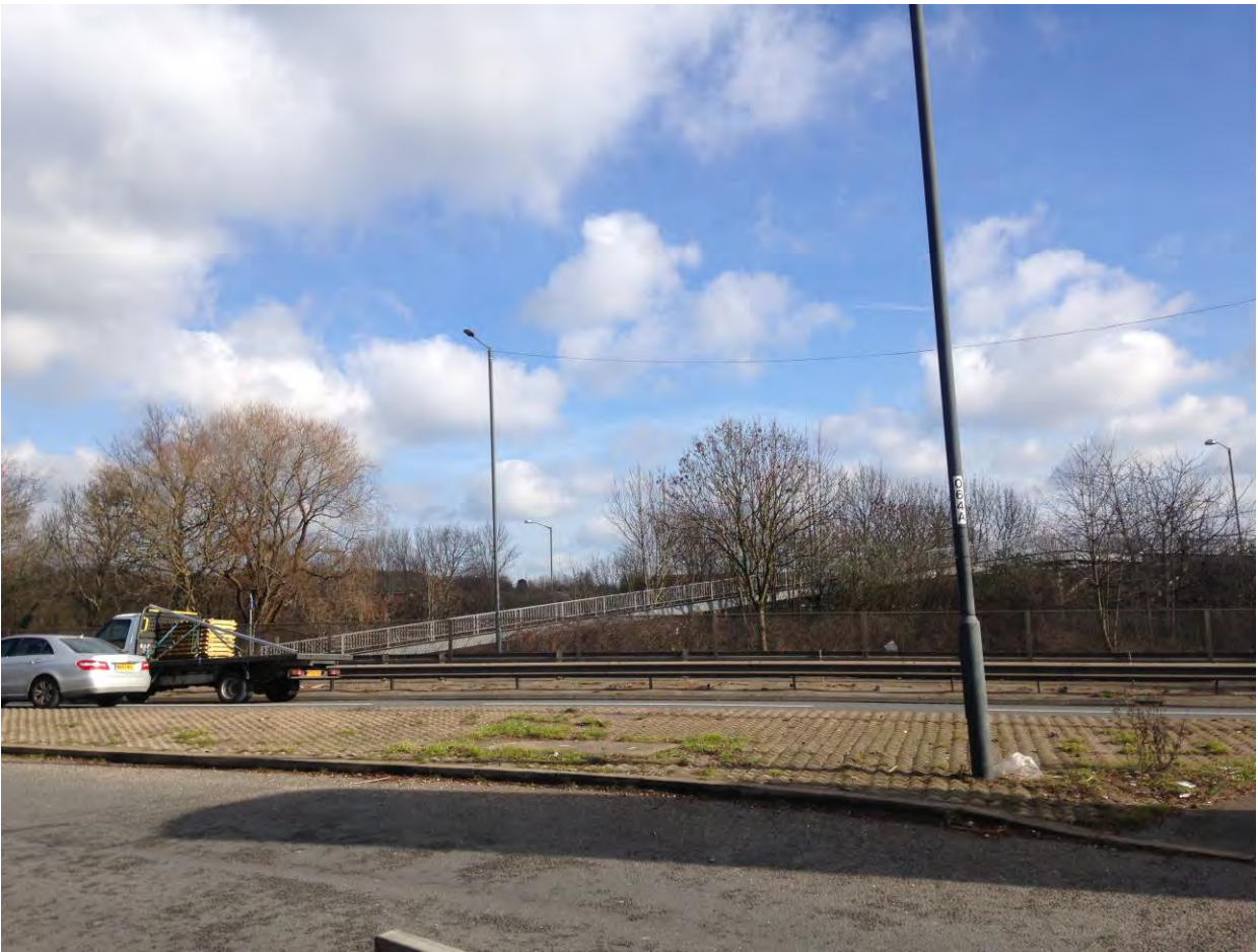
Figure 18: View east from the eastern boundary of the Site, towards the elevated pedestrian crossing over Watford Way.
