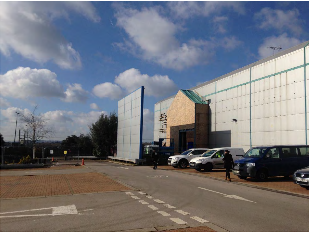
Figure 23: View west from the centre of the Site towards partially demolished warehousing
