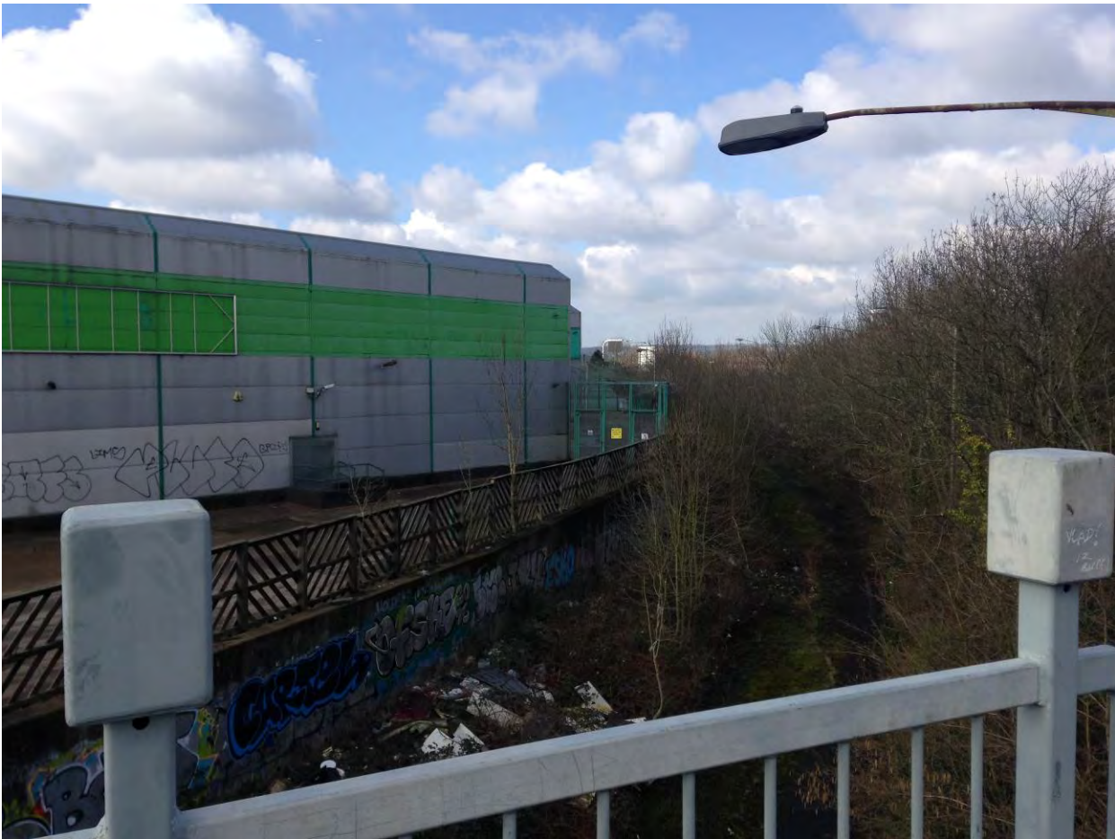
Figure 16: View from pedestrian access to the Site from Watford Way. The derelict nature of the Site is evident from this view.
