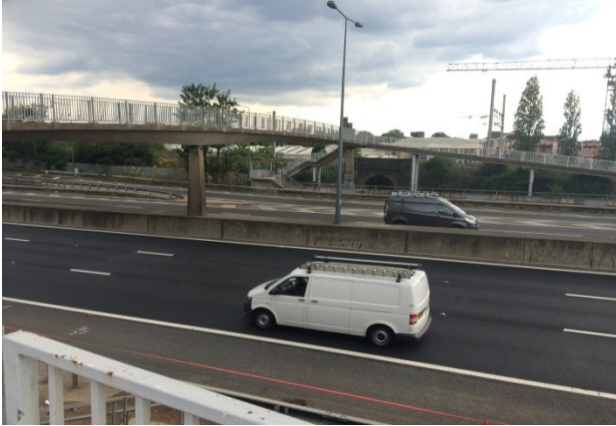
Figure 9: Pedestrian bridge over M1
