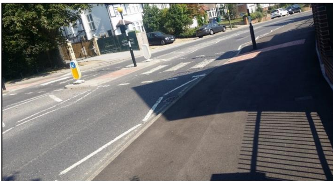
Figure 3-2: Zebra crossing on Bunns Lane
