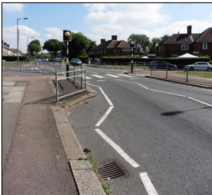
Figure 3-1: Zebra crossing on Watling Avenue
