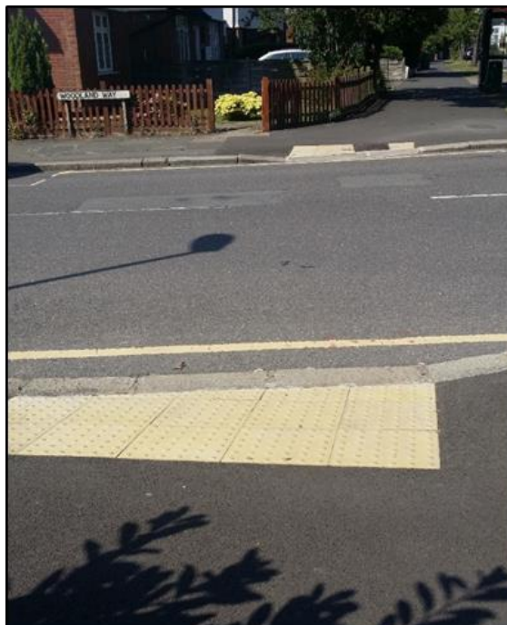
Figure 3-4: Uncontrolled Crossing on Woodland Way
